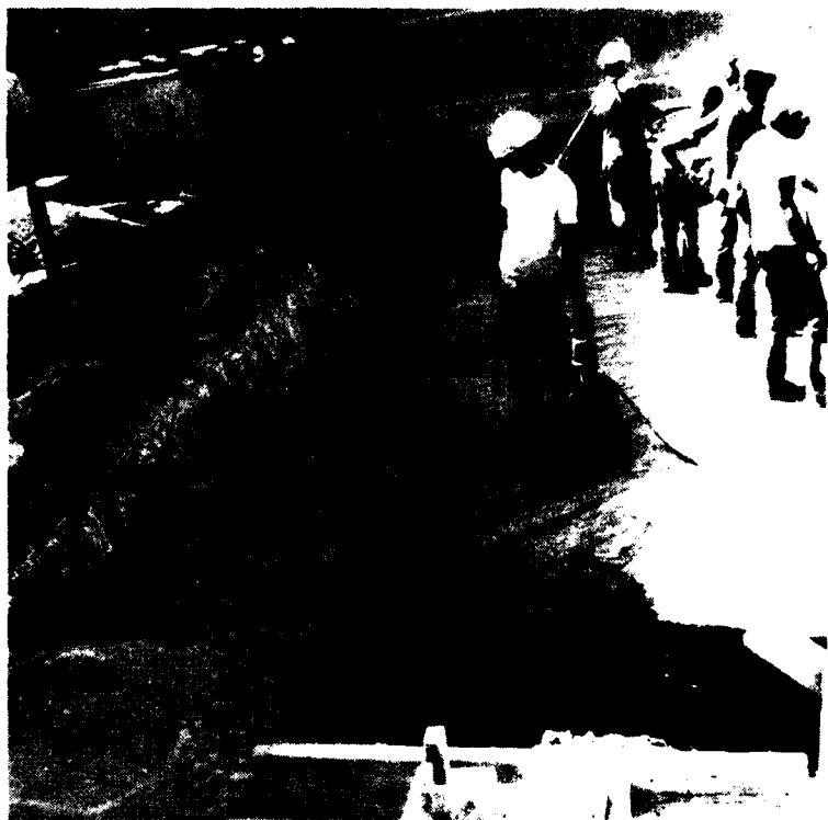
Station 4+65, Offset 205-215 feet downstream, view north, applying bituminous coating on final foundation of Stilling Basin. 17 June 1976
