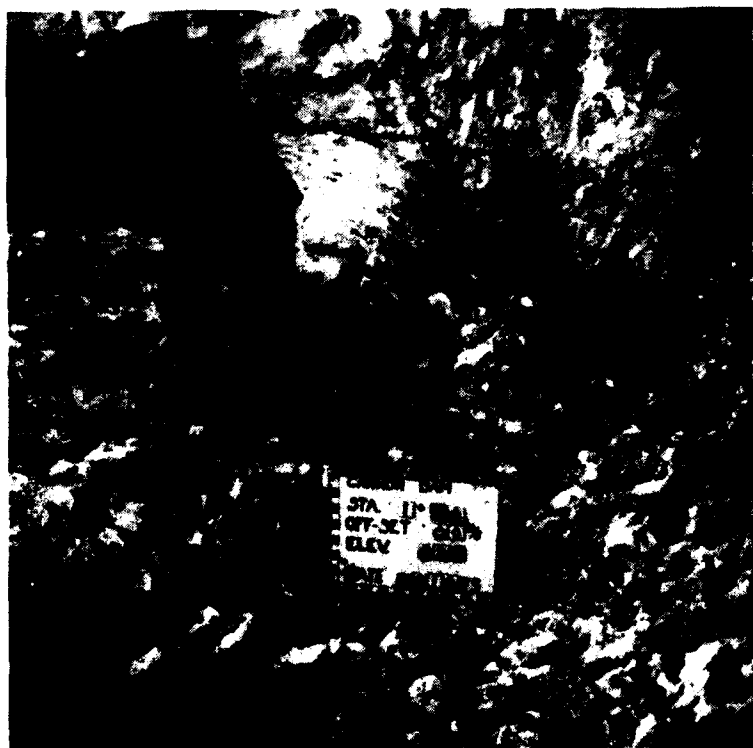
Station 1+38, Offset centerline, Elevation 626 feet. Final foundation preparation of collapsed sinkhole in Monolith D17. 13 October 1975.
