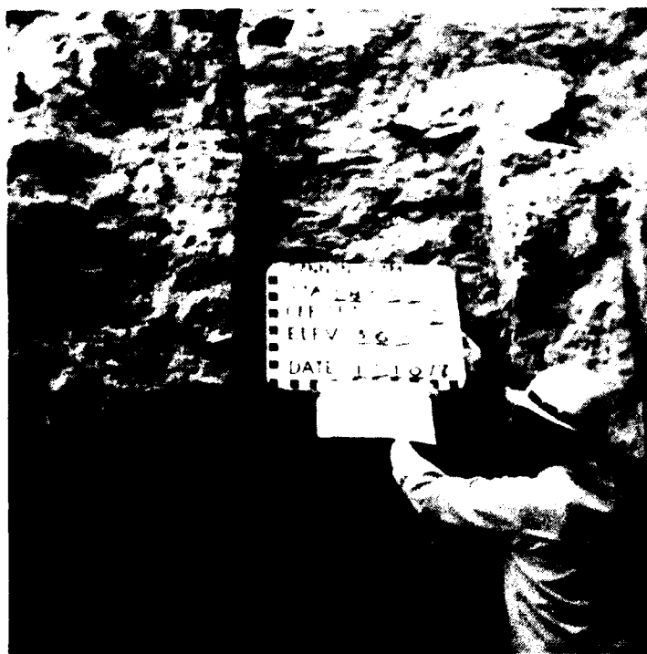
Cutoff wall, final foundation for concrete placement CW 5-2. Station 18+58, Offset upstream, Elevation 560-570 feet. 10 Oct. 1978.
