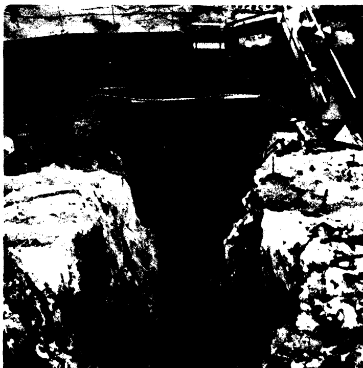
Left abutment cutoff wall. cavity #1. Looking down from top of cutoff trench into cavity, base of cavity elevation 600 feet. 12 Oct. 1978.
