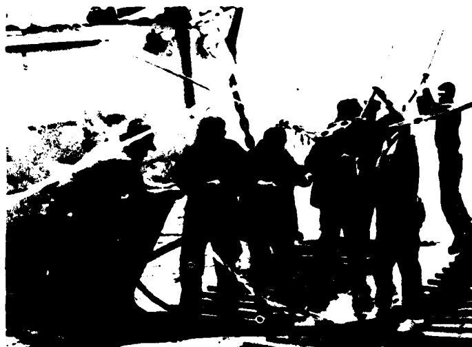
Seabees placing protective pipe on underwater cable
