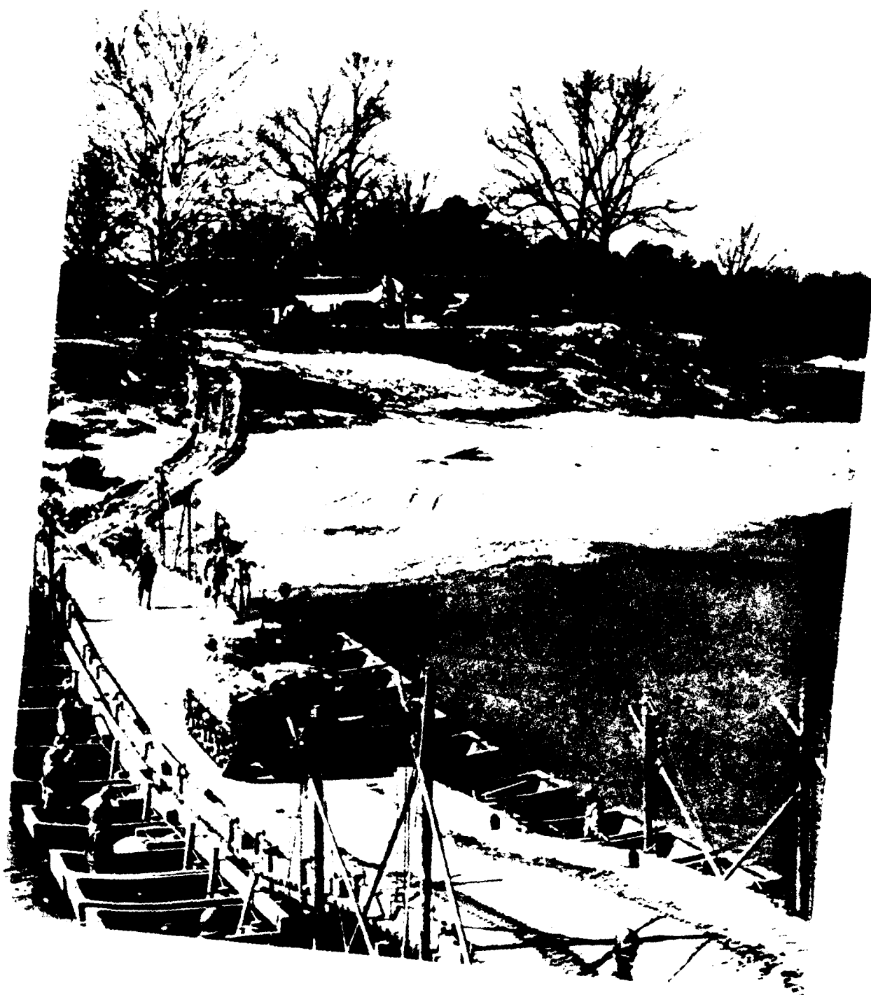
... so that tanks could cross a few hours later ... 741st Tank Bn. crossing the Sabine River at Haddon Ferry over a pontoon bridge built by the 180th Eng.
