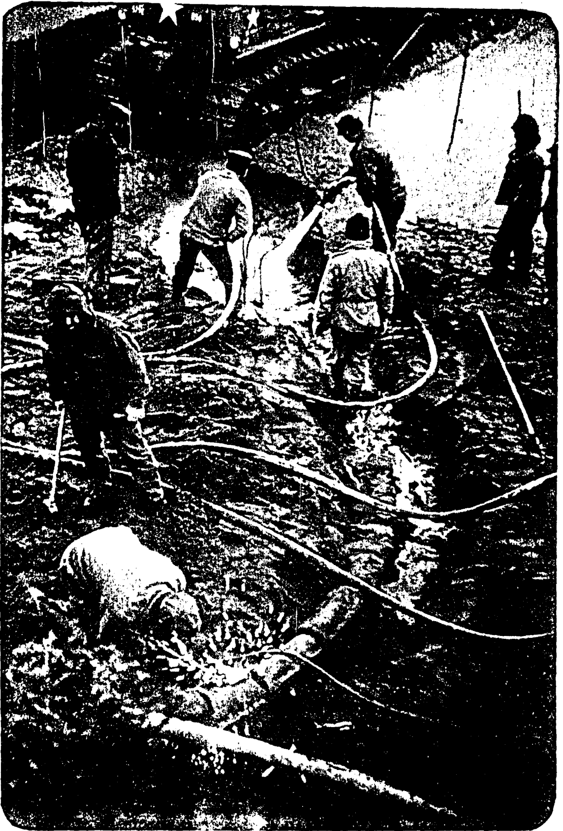
Men working on the cable.
