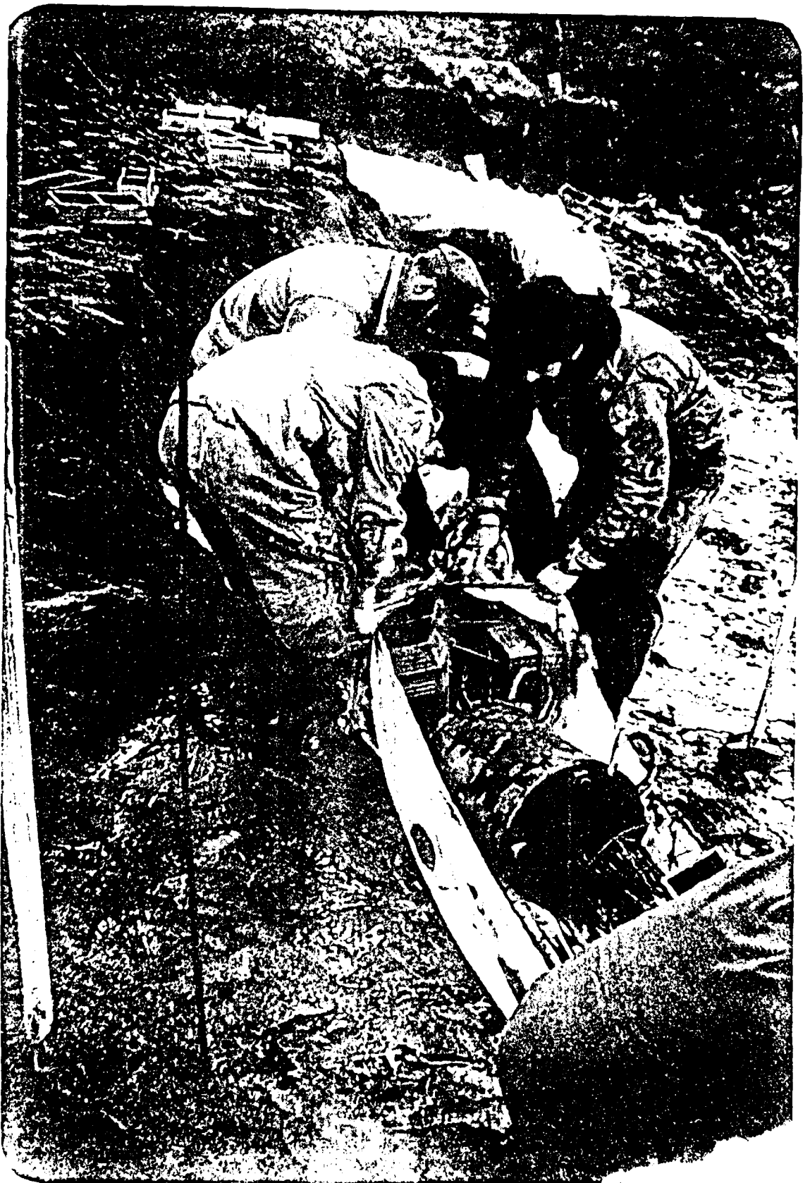
Figure 11. The men working in the trench.
