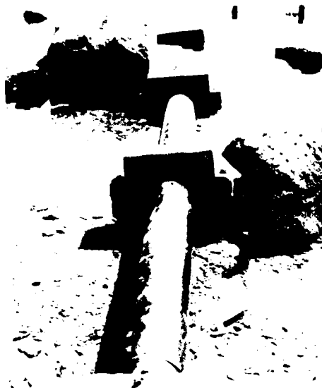
Outfall No. 31 the outfall is intact
