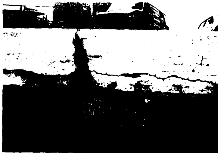
23. Bulkhead # 1. Picture shows horizontal crack caused by rusting reinforcing steel near Station 0+00.
