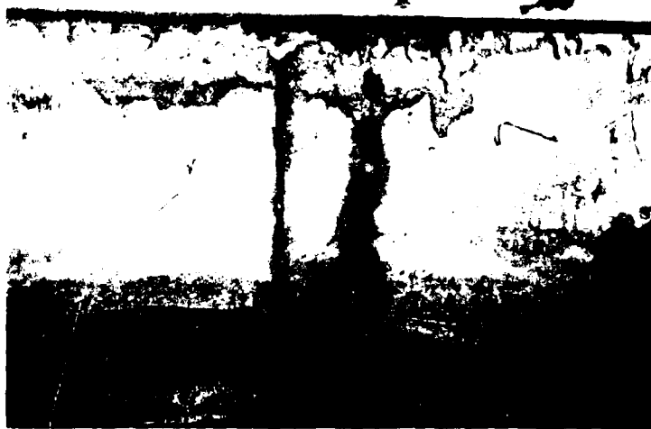
24. Bulkhead # 1, near Station 0+00. Picture shows typical bleeding vertical crack in precast panel.
