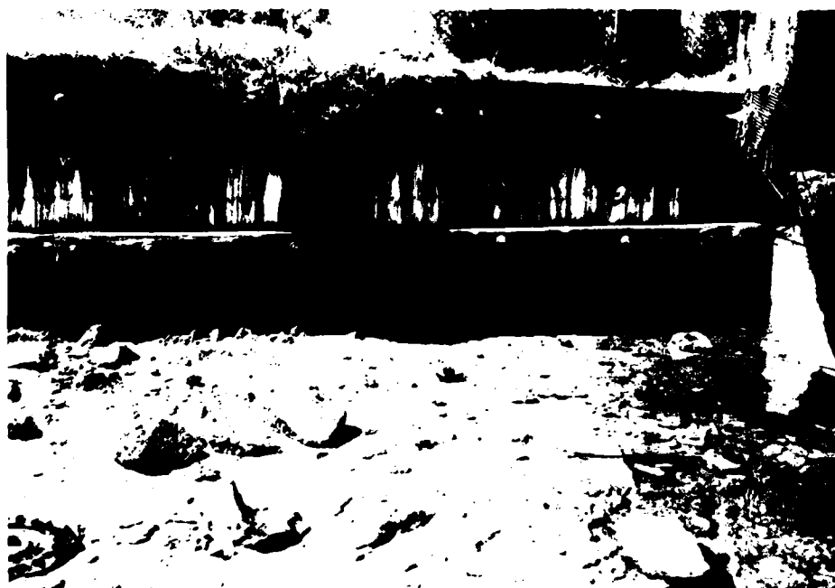
20. North Boundary Bulkhead. A closer view reveals the deterioration of both wales and lagging. The wall apparently is stable due to tie-back rods extending to dead men anchors in the backfill. This is evidenced by the large square washer connections seen at the lower wale.
