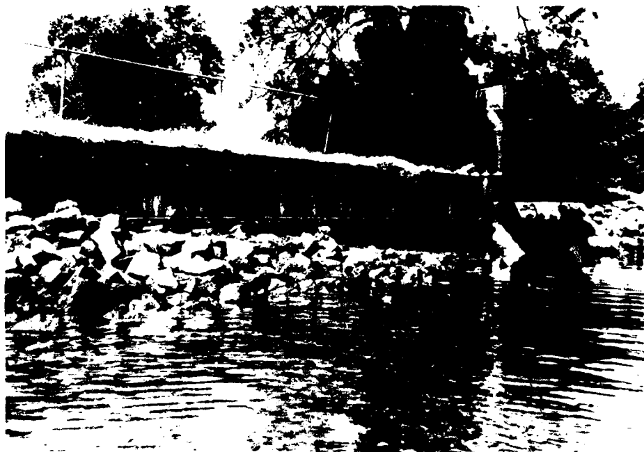
19. North Boundary Bulkhead. Fence in the right foreground is the boundary with Marine Corps Recruit Depot. The wood has deteriorated from dry rot.
