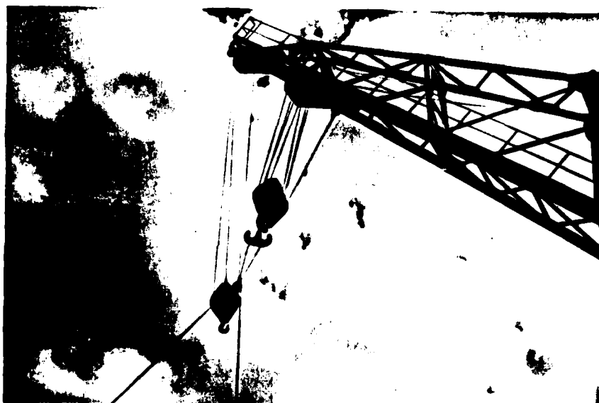
DAMAGED CRANE BLOCK ASSEMBLY ANCHOR STILL SUSPENDED
