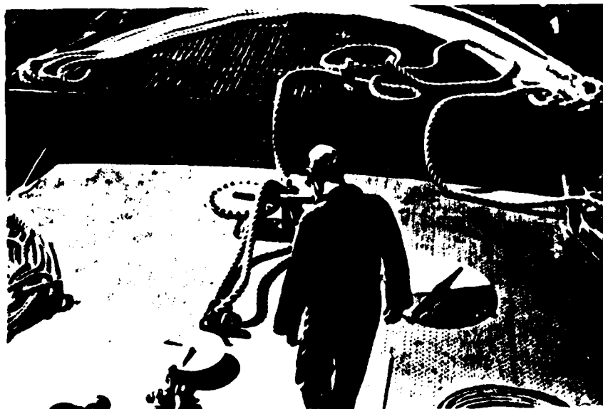
RIGGING DYNAMOMETER FOR PULL TEST ON MOORING BUOY #5
