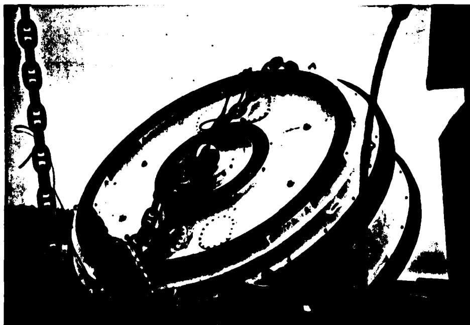
THROW-OFF LEGS BEING SECURED TO MOORING BUOY
