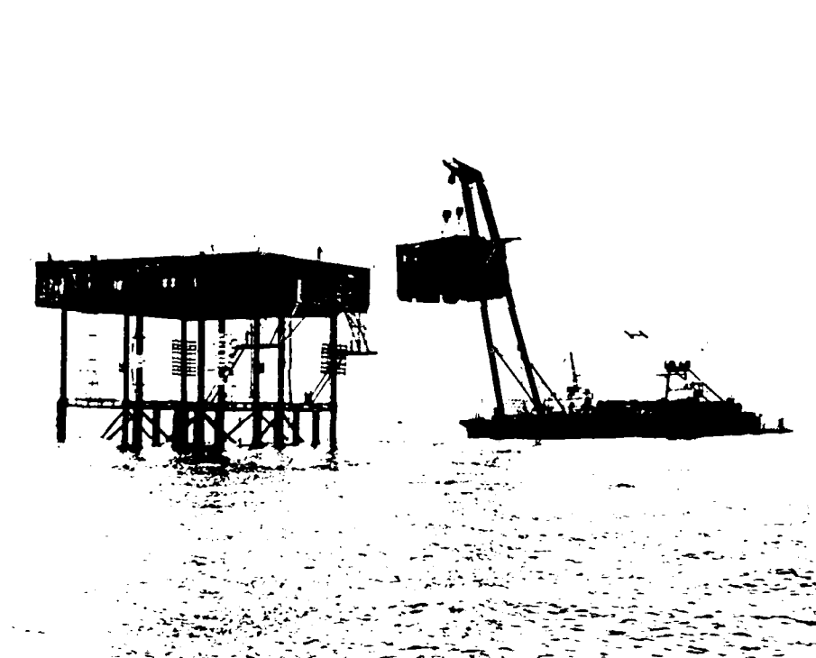
Figure 28. Section I (Upper Two Decks) Being Removed from Stage II (5 August 1984, weight = 60 tons)
