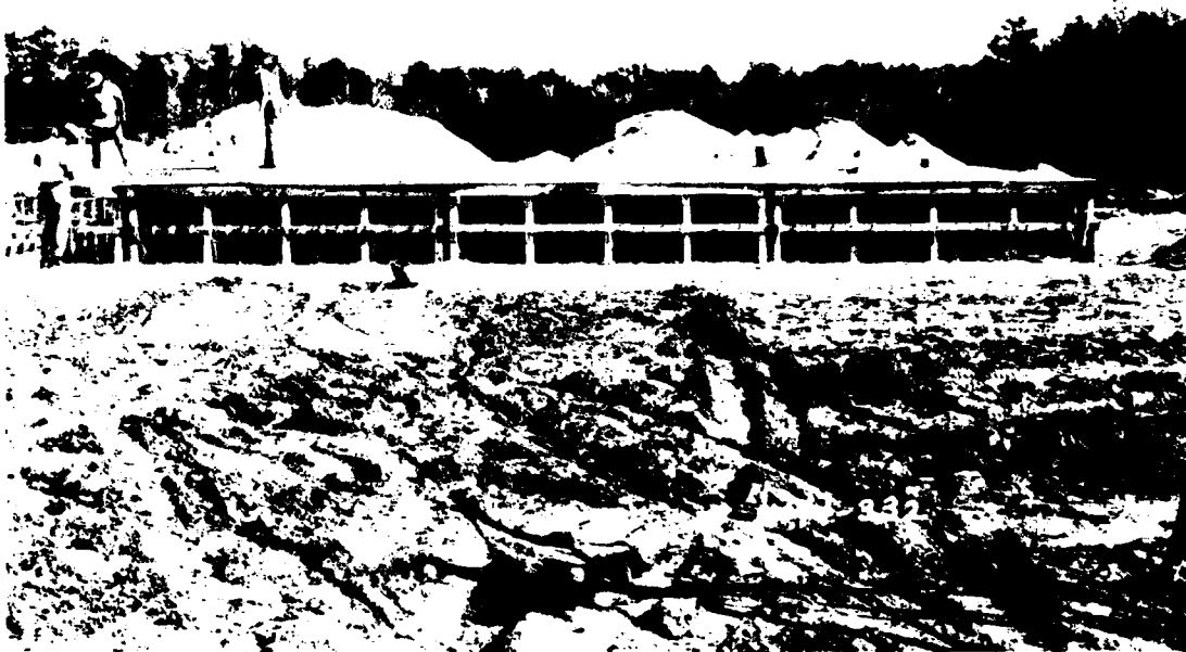
Figure 2.7. Charge cavity construction.
