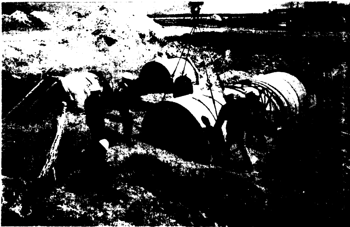
Figure 16. Arch A5-1 placement.
