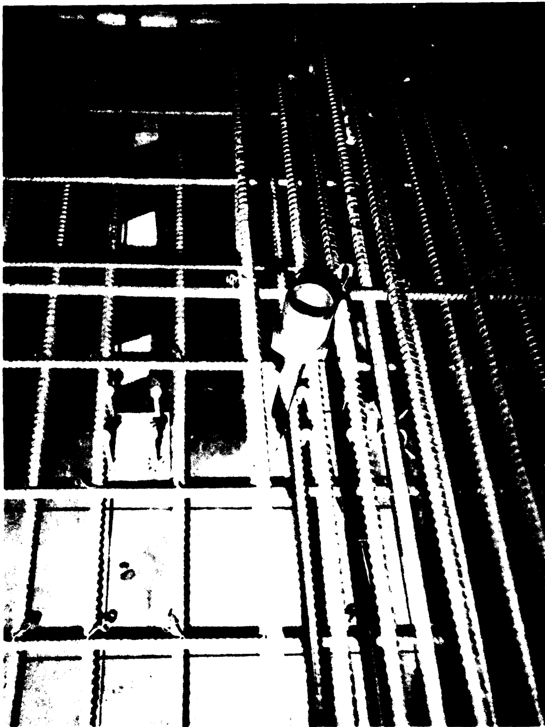
Figure 5. Cast-in-place instrumentation hardware.
