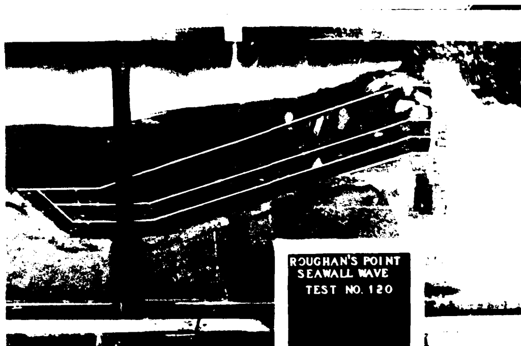
Figure 9. Configuration 2, seawall with standard riprap revetment as it appeared in the model study
