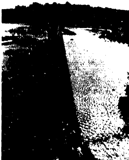
Figure 18. The Lake Brownwood emergency spillway. The unlined discharge channel is immediately downstream (to the right in this view to the northeast) from the 480-ft-long broadcrested weir
