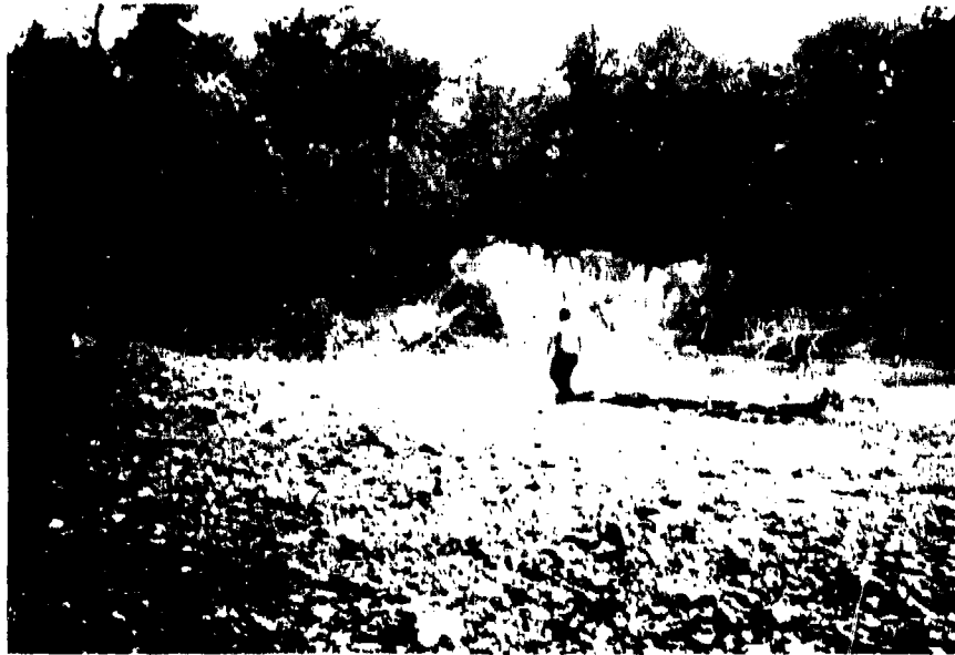
Figure 45. Gravel fan formed by spillway overflow at Wister Dam (SWT) Tulsa District. Formation forced flow against outer channel bank causing bank erosion
