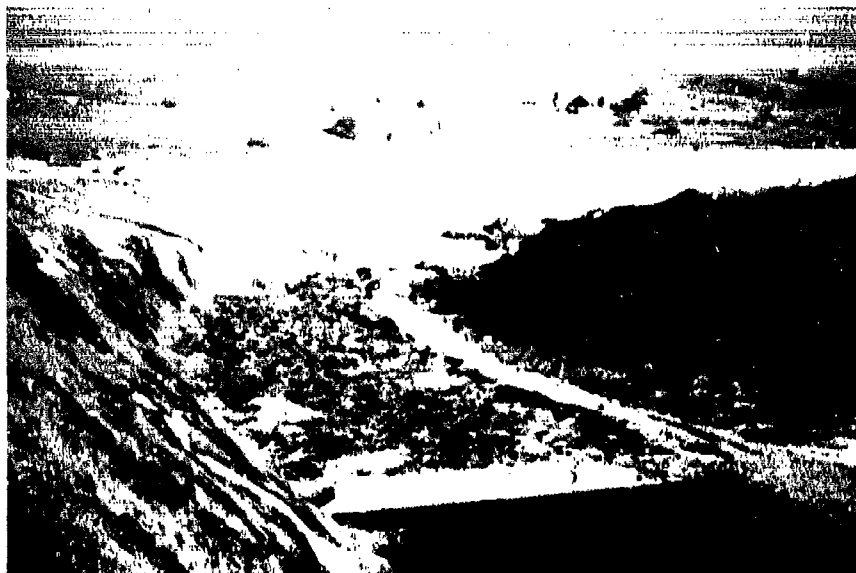
Figure B1. Downstream view of eroded Black Butte spillway following 1983 overflow. The spillway floor is composed of basaltic and pyroclastic materials. The reinforced-concrete spillway weir is in foreground. The linear structure, right center, is a road used to haul materials for remedial dam work several years before overflow
