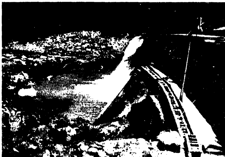
Figure 41. A 30-ft waterfall now occupies the site of the failed downstream spillway apron at a private reservoir on Johnny's Creek near Fort Payne, Alabama. Excessive scour undercut the concrete structure during an estimated 100-year storm in the summer of 1985
