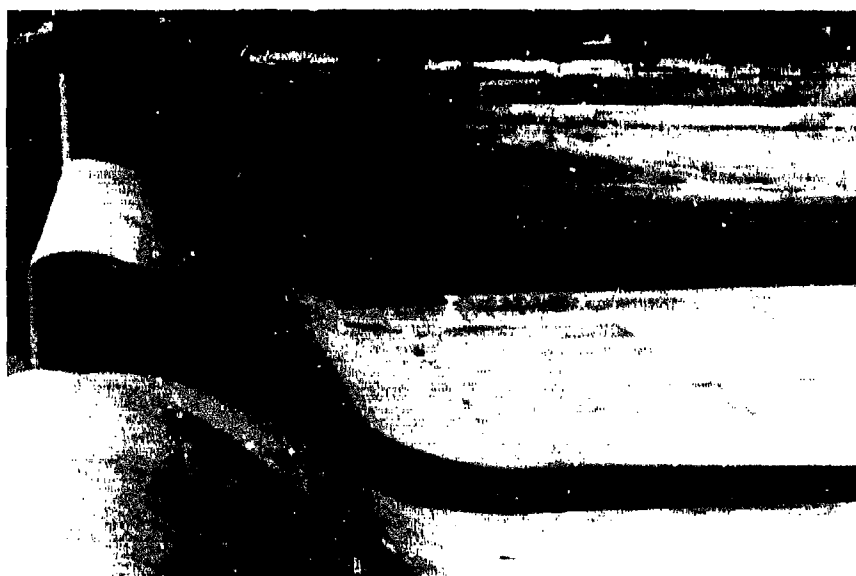
Figure B3. Notched ogee spillway weir at Benbrook Dam, Texas
