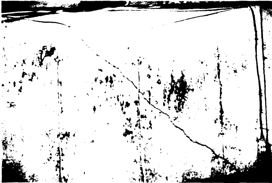
Figure 12. Photograph of cellar of house on Old Payson Road, Northfield, New Hampshire showing crack in poured concrete wall.
