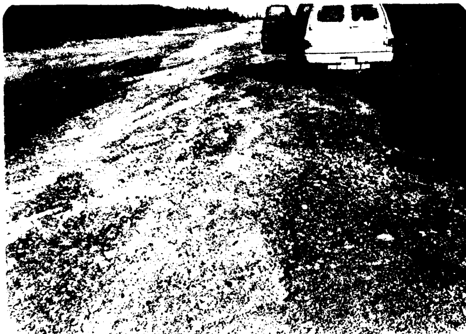
b. North site, looking north along the west shoulder. Note the shoulder cracking and the service road adjacent to the runway.
