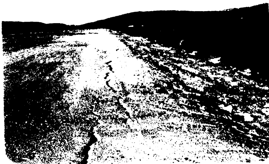
b. East site, looking west from the cross section along the north side of the runway. Note the cracks along the runway edge, probably caused by the settlement at the toe area. Also note the surface water along the toe.
