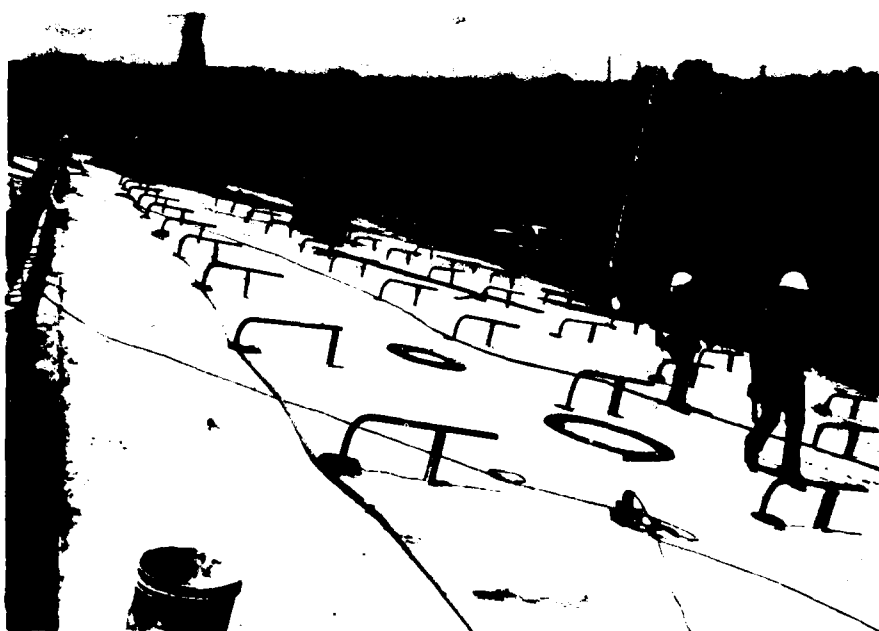
Fig. 8 - Anchor bars in place and ready for grouting
