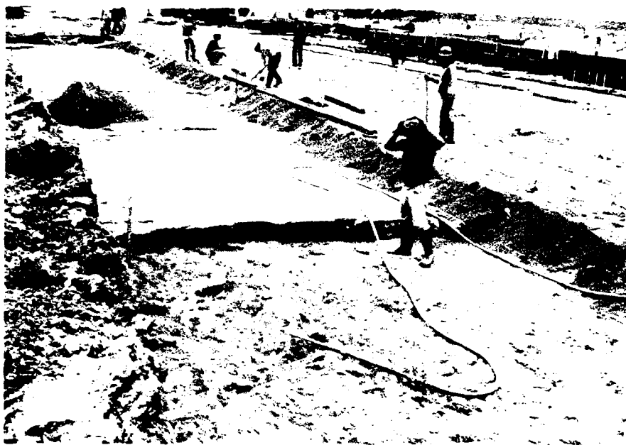
Fig. 30 - Exposed foundation surface - 6 March 1985
