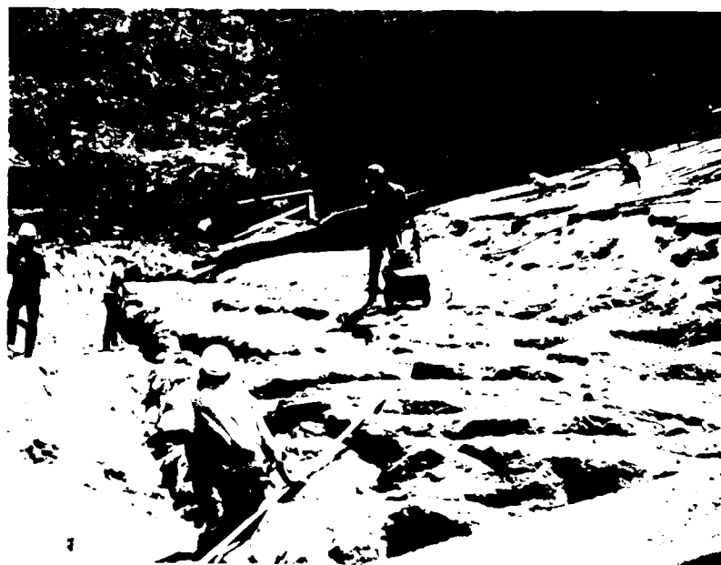
Fig. 25 - Exposed foundation surface - 17 September 1984
