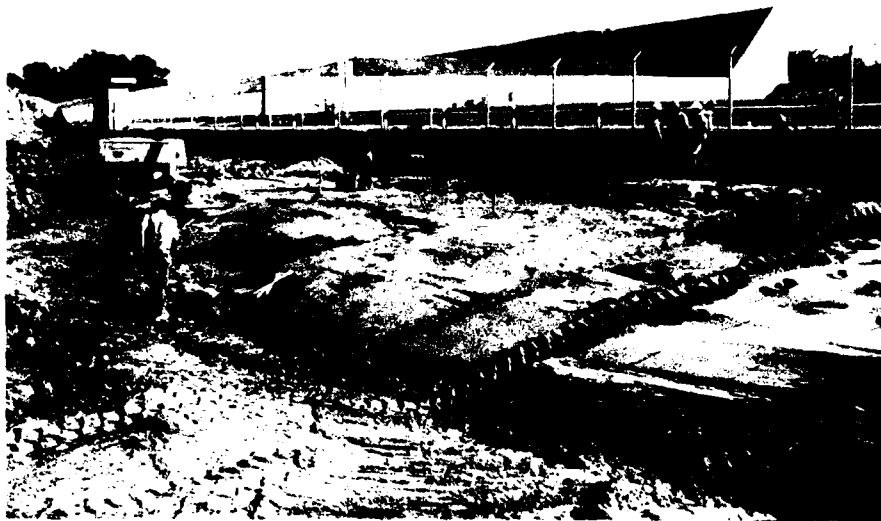
Fig. 14 - Exposed foundation surface - 25 April 1984
