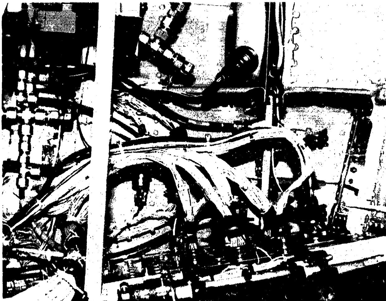
Figure 98. Wire Routing Through Cockpit Bulkhead Connectors
