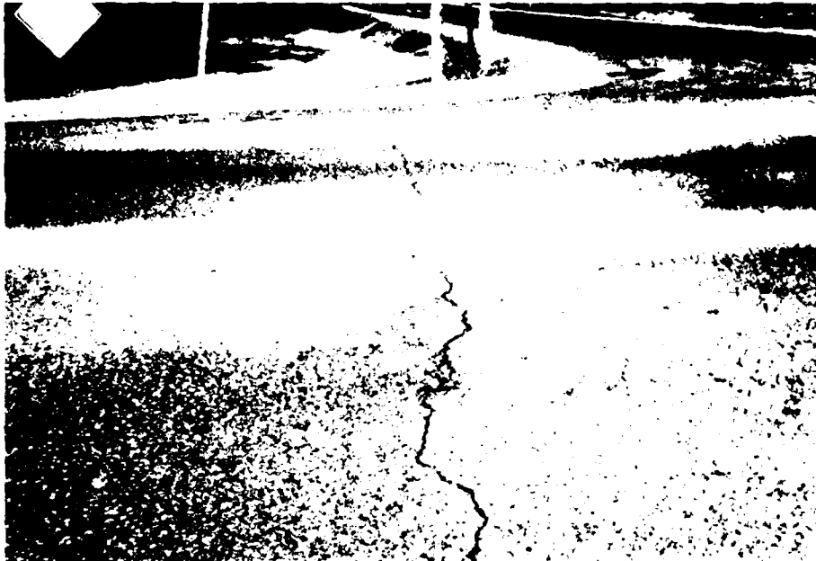
Figure 21. Typical transverse crack over original AC pavement, US 2, Spokane County
