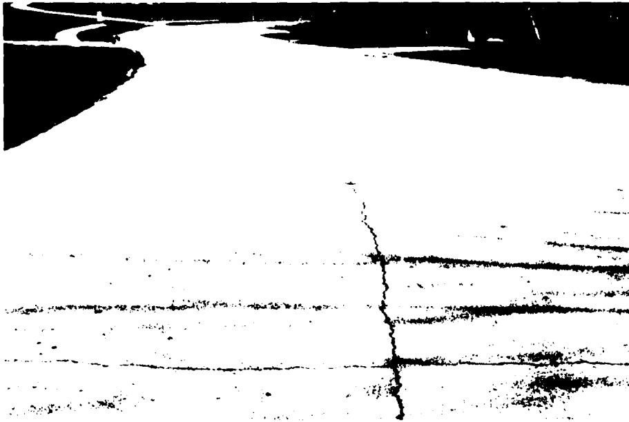
Figure 22. Longitudinal crack in engineering fabric section, Cottage Grove Road, Urbana
