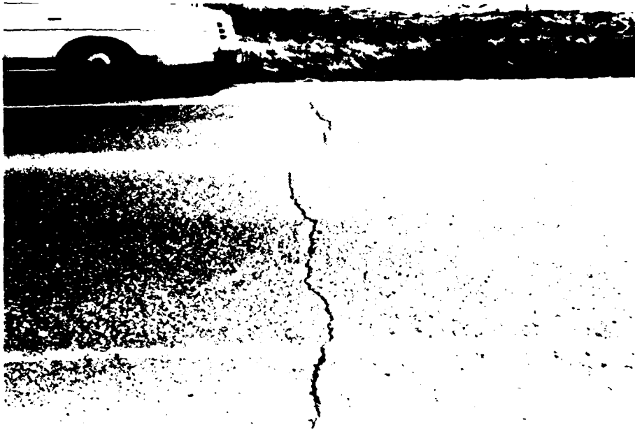
Figure 20. Typical transverse crack over original PCC pavement, US 2, Spokane County
