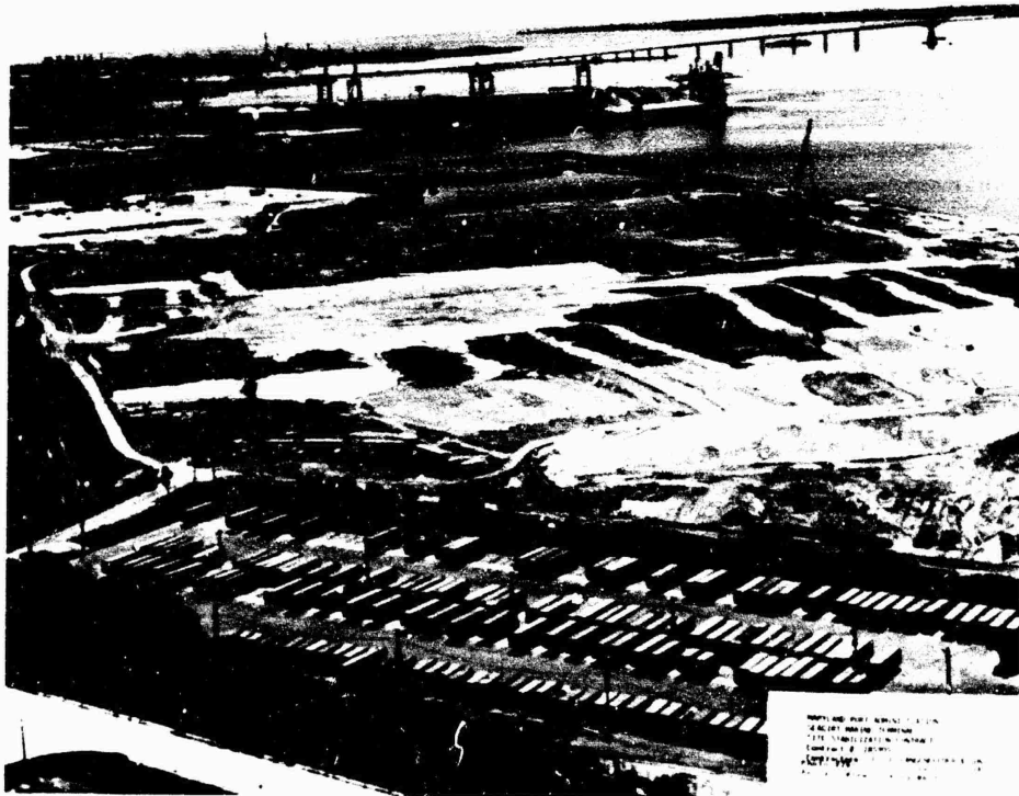
Figure 18. Aerial view of MPA's "Seagirt" stabilization project
