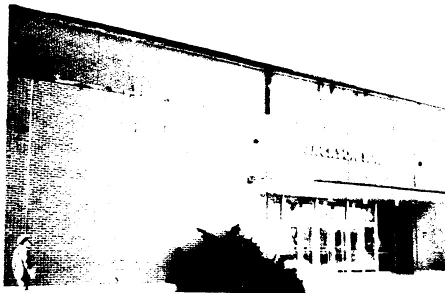
Figure 4. Building selected for PVC roofing at Chanute AFB.
