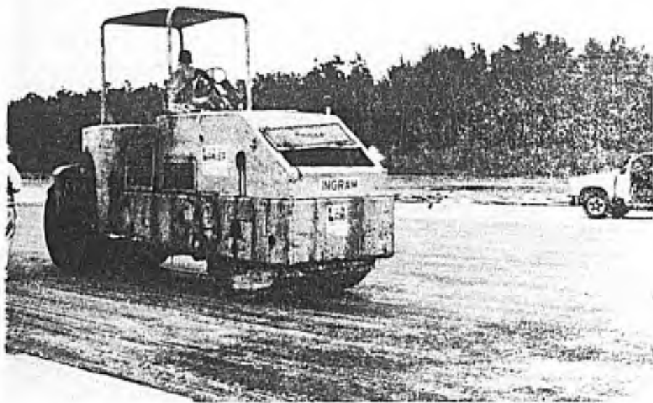
Photo 19. Final Compaction of the AC with a Tandem Steel-Wheel Roller.
