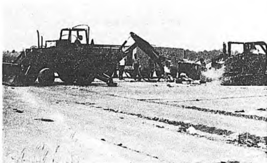
Photo 4. Removal of PCC With Pavement Breaker and Front-end Loader.
