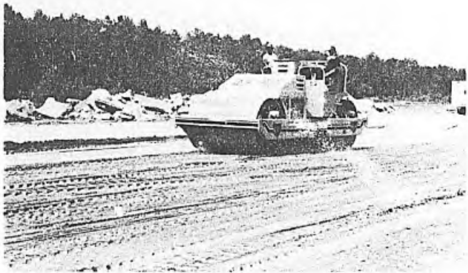
Photo 5. Compacting the Subgrade With a Tandem Vibratory Roller.
