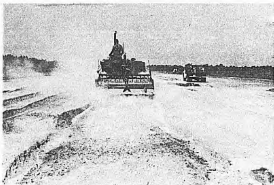
Photo 9. Blending PC and Silty Sand with a Pulvimixer.
