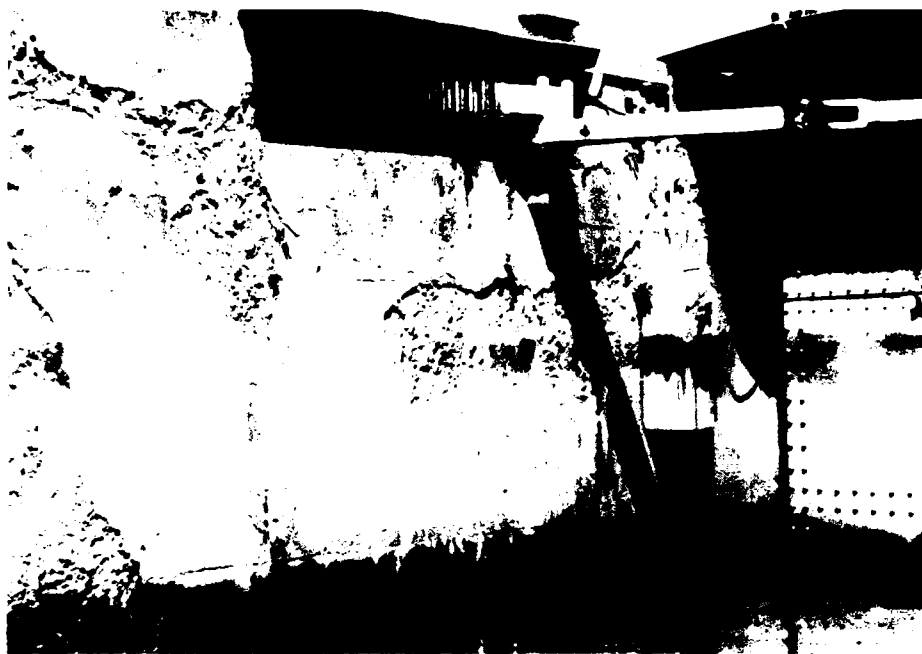
c. Lower miter gate recess, land lock wall, showing spalling, scaling, and some evidence of leaching
