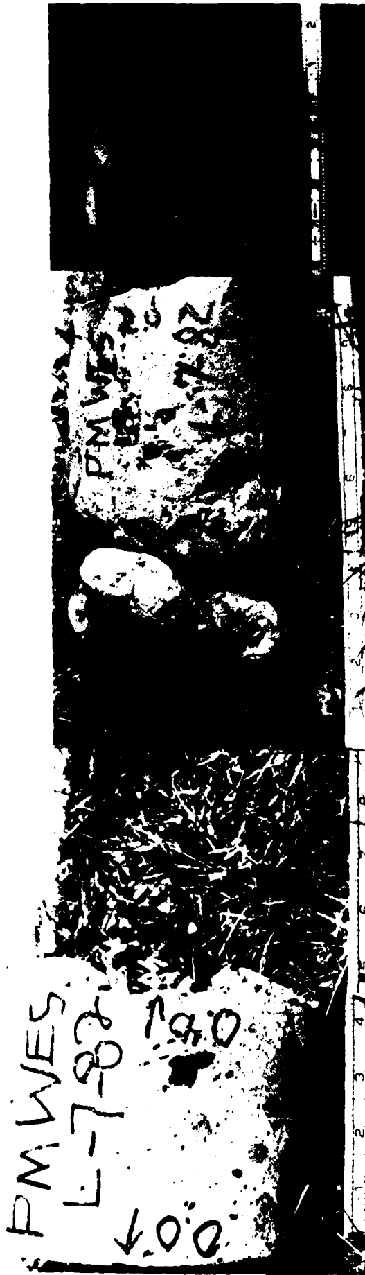
Concrete core, boring L-7-82, overlay concrete, 0.0 to 0.45 ft, missing rubble and cracked concrete to 2.5 ft
