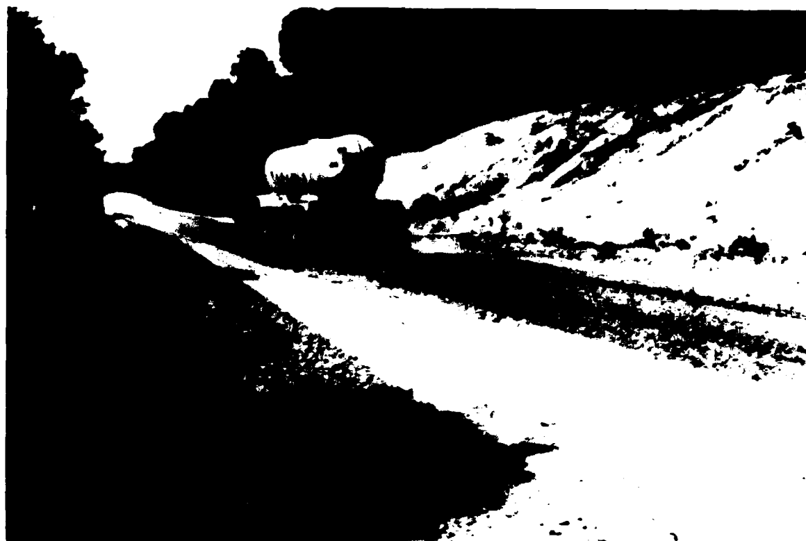
Figure 10. Application of brine solution with adjustable spray bar
