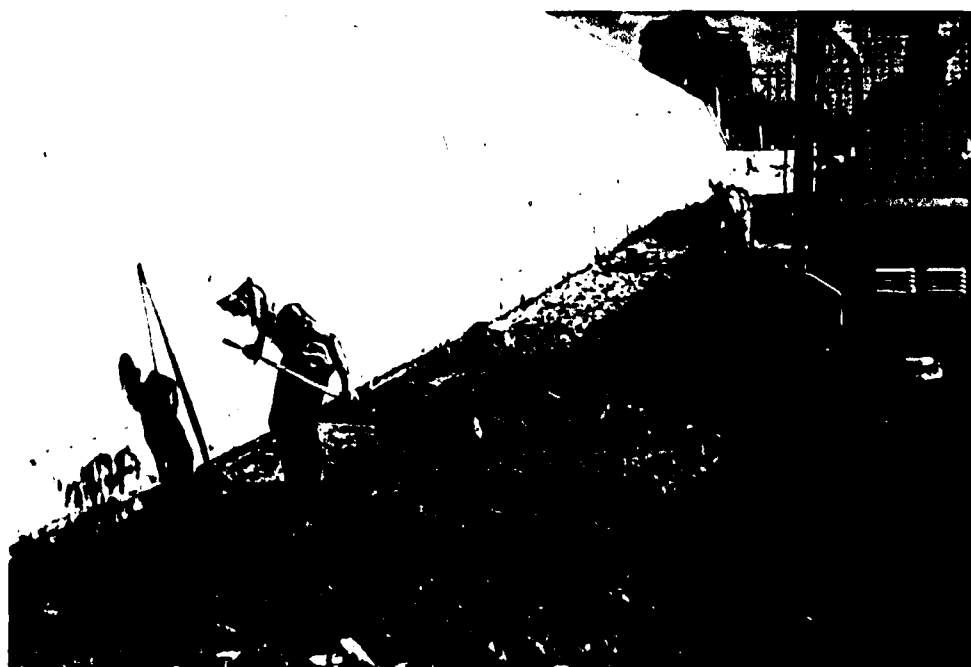
Longview Lake, 1 Jun 81, Neg. No. 706. O.W. Station 52+35 on right side. Look downstream. Foundation cleanup. Pleasanton Formation zone 1.
