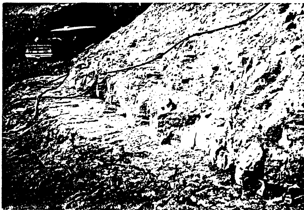
86. Longview Lake, 19 Mar 81, Neg. No. 591. Station 87+85 right abutment look at downstream corner of cutoff trench. Bethany Falls Limestone and Hushpuckney Shale.
