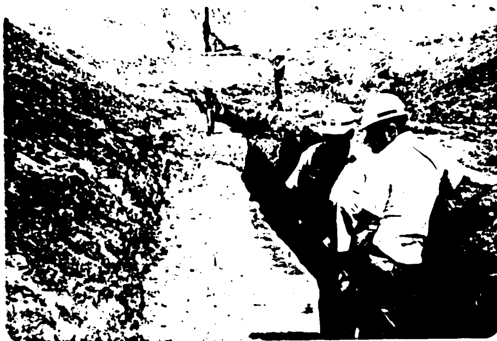
65. Longview Lake, 10 Jun 80, Neg. No. 22. Cutoff trench Station 90+70, range 10' ± D/S. Look southeast. Preparing for placement of pervious drain.
