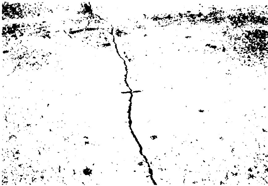
Photo 13. Typical unsealed, low-severity cracking, main taxiway (T13A)
