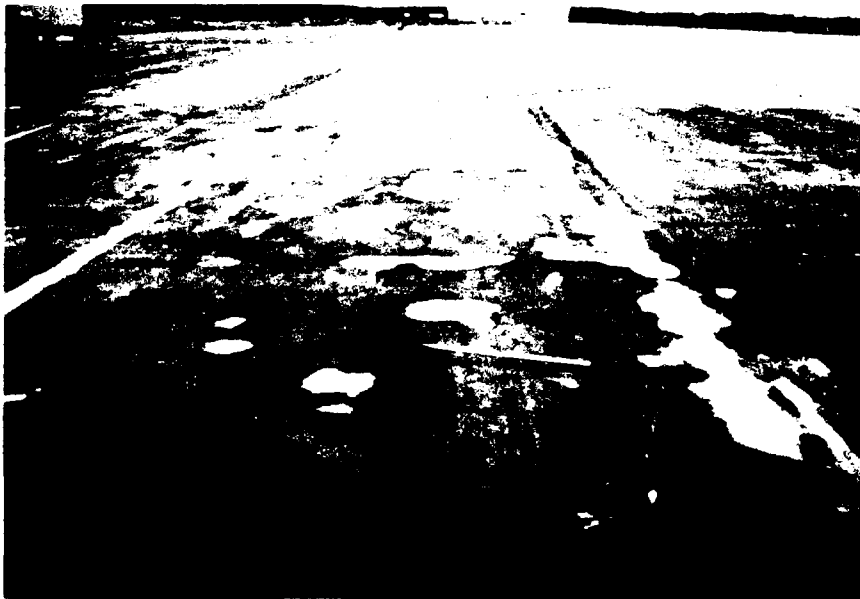
Photo 30. General view of fuel pit area and low-severity rutting, south apron (A11B, Section 3)
