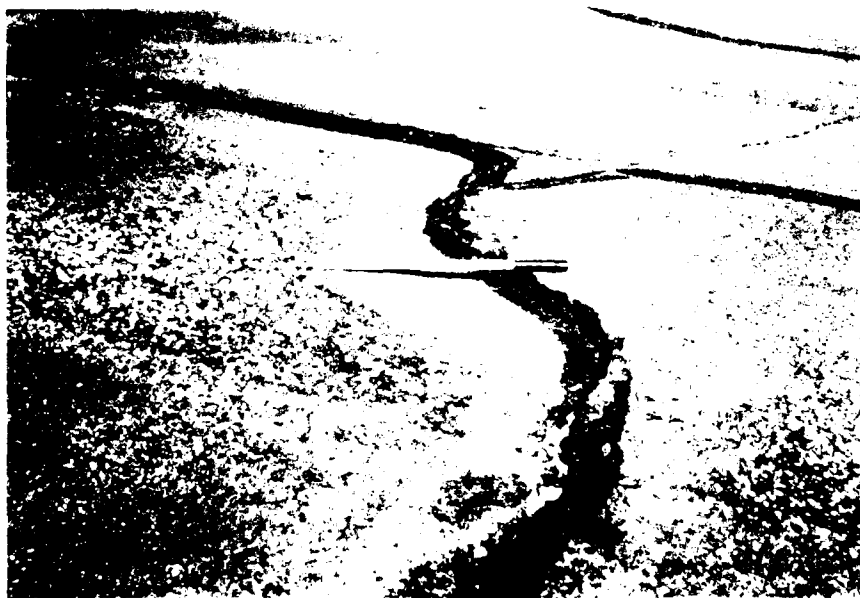
Photo 24. Faulted high-severity crack, C-135 apron
