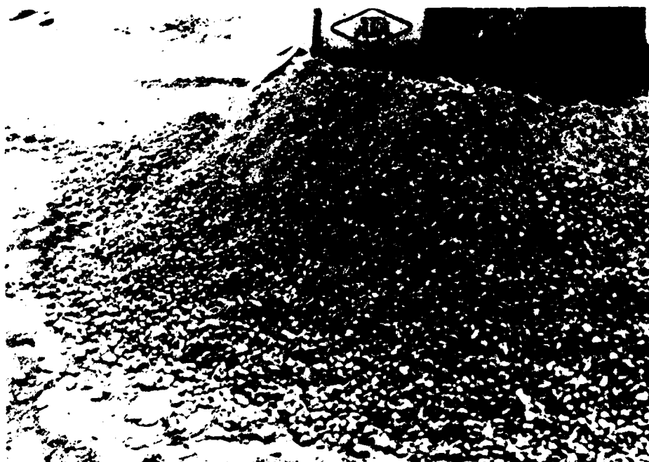
Photo 28. Dumping concrete directly onto prepared base. (Notice some segregation)
