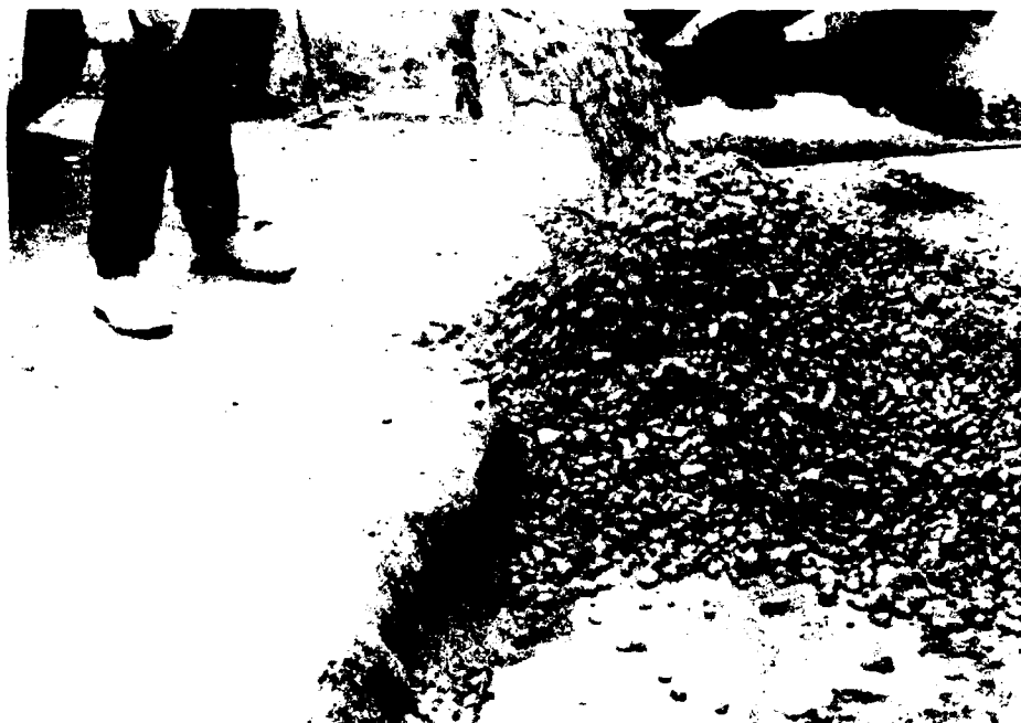
Photo 31. Placing RCCP along the vertical edge, Item E
