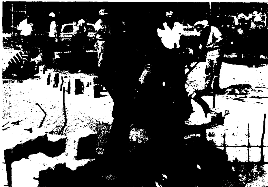
Photo 51. Cutting paving blocks with a hydraulic rock splitter
