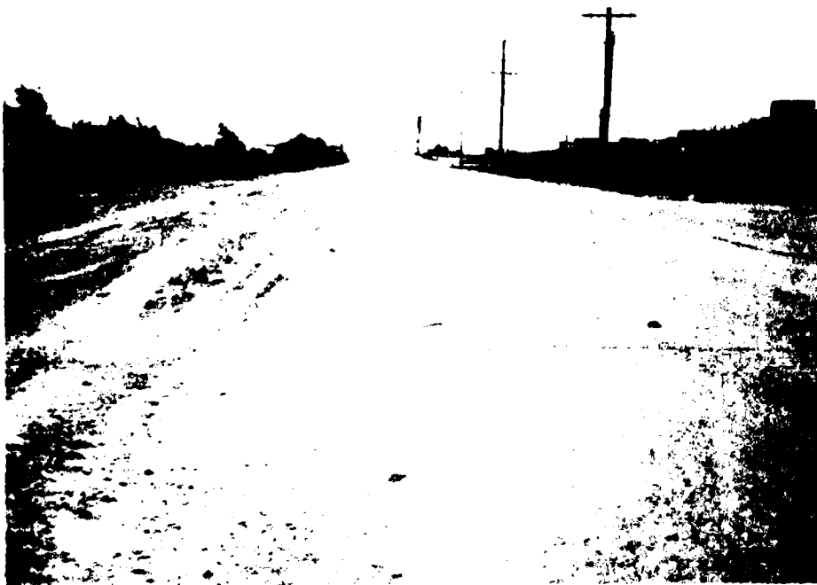
Photo 2. Rounded pavement edge caused by tracked-vehicle traffic, Fort Hood
