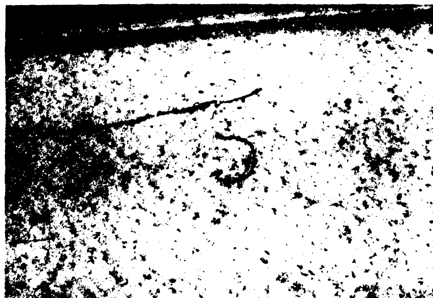
Photo 60. Root pulled from latex asphalt concrete surface
