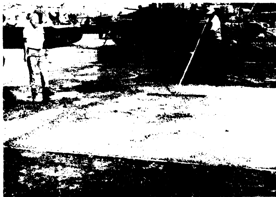
Photo 18. Floating the surface of Item A, FRC
