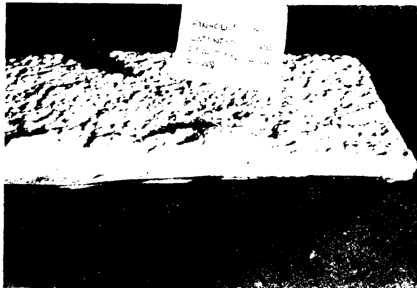
Figure 32. Foam application over wet surface.
