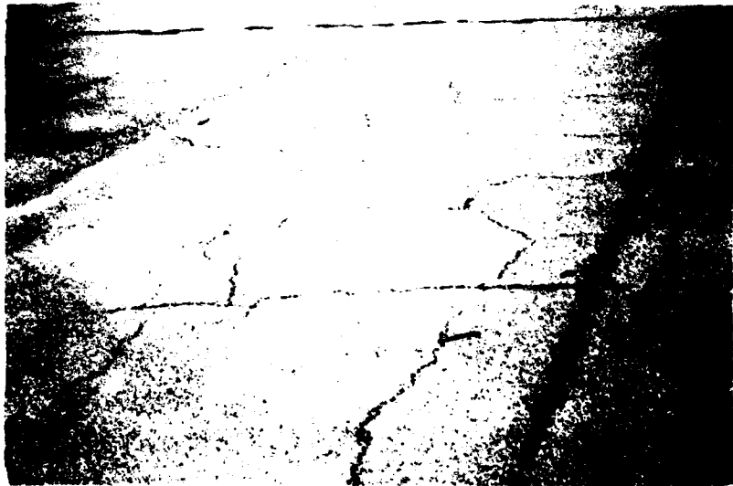
Photo 19. High severity joint reflection cracking and medium severity block cracking, south ramp
