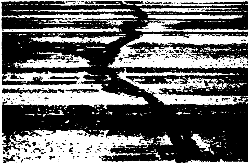
Photo 1. Medium severity cracking in PCC, Runway 4-22 (R3B)
