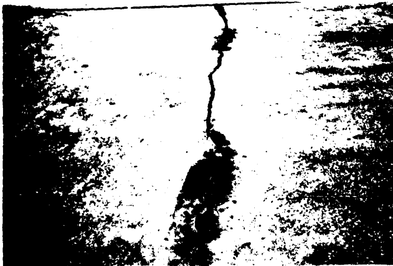
Photo 2. Sealed, low severity crack, Runway 4-22 (R5B)
