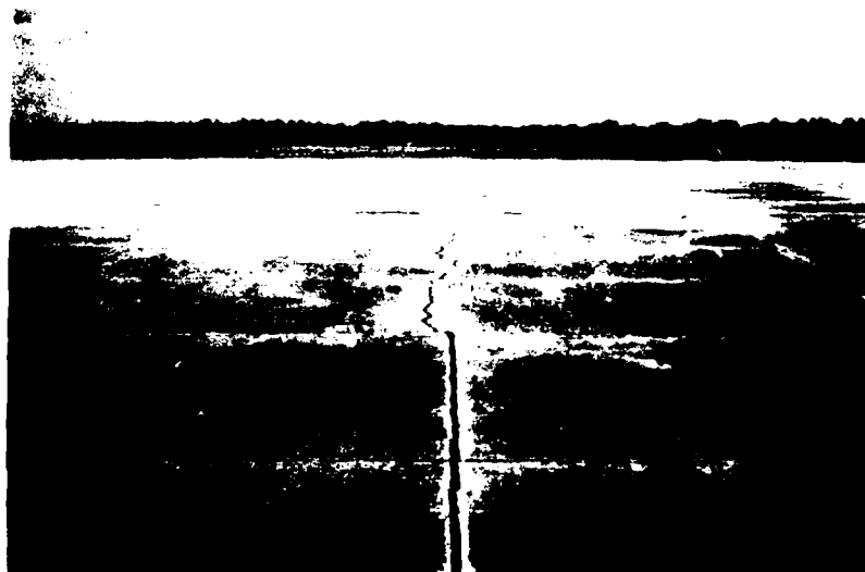
Photo 5. View of cracking caused by uncut joint, Apron E
