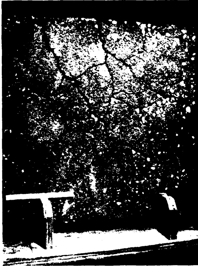
Figure 1. Typical "cracked" concrete slab.
