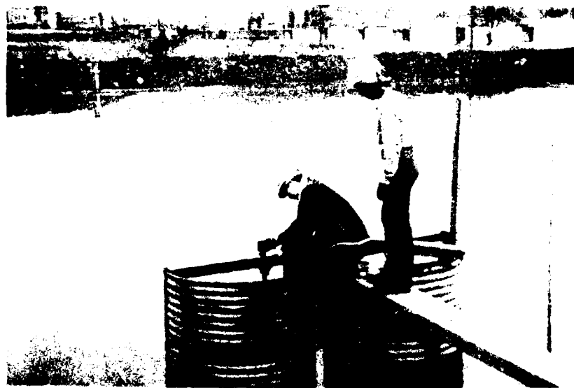
Figure 26. Drop inlet weir structure, Black Rock Harbor field evaluation
