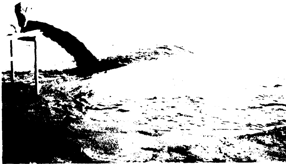
Figure 17. Influent pipe, Norfolk Harbor field evaluation
