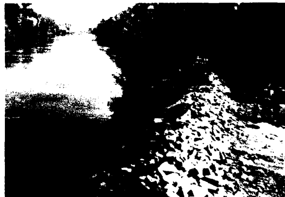
Rubble revetment constructed from broken pavement, concrete blocks, and house brick.
