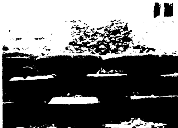
Stacked tires should be packed with stone or rubble.
