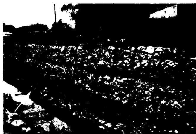
Completed gabion revetment made from prefabricated baskets. Note support apron (arrow) extending from toe of structure.
