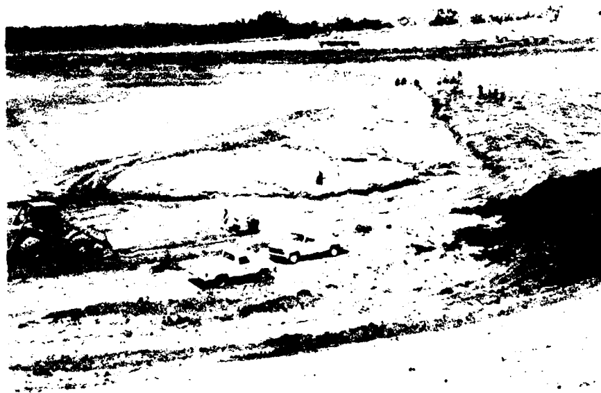
Figure 10. Excavation slope being prepared for backfill. Right (north) side of right abutment deep inspection trench. 2 September 1982.
