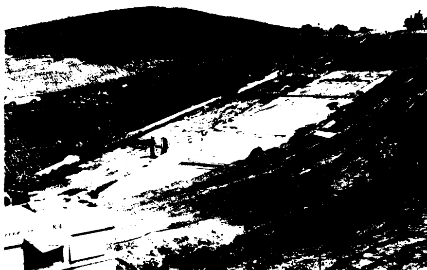
Figure 40. Spillway foundation being prepared for backfill with sand filter blanket and protective slab. 9 April 1983.
