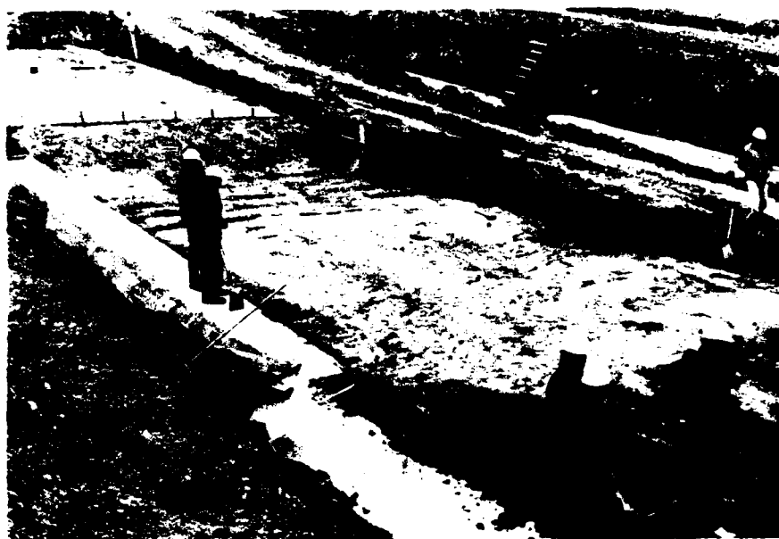
Figure 42. Spillway foundation being prepared for backfill with filter blanket and protective concrete. 5 April 1983.
