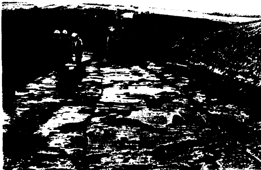
Figure 11. Excavation slope being cut to final grade. 20 November 1982. Photo taken at right abutment deep inspection trench, station 10+50, looking west.
