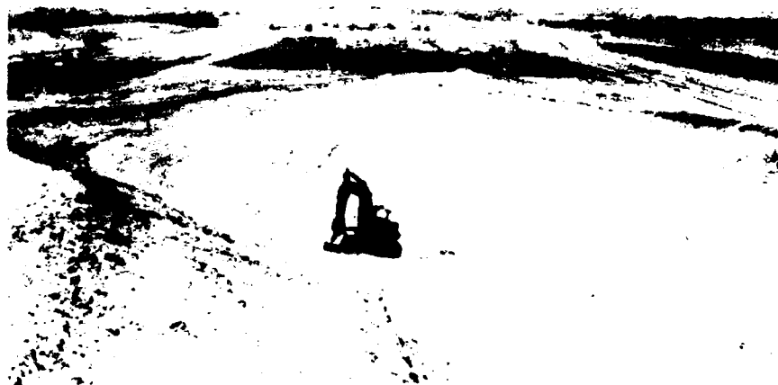
Figure 5. Right abutment deep inspection trench after completion of bulk excavation and prior to start of final surface cleaning and backfill. Photo taken at embankment station 8+00, looking west.
