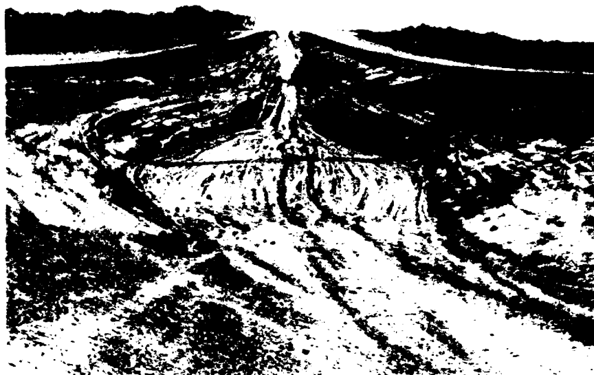
Figure 6. Right abutment deep inspection trench after completion of bulk excavation and prior to start of final surface cleaning and backfill. Photo taken at embankment station 18+00, looking east.
