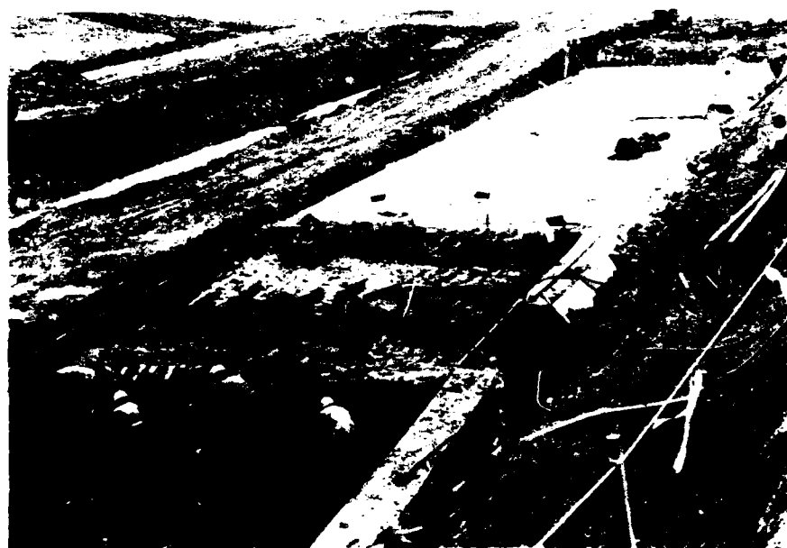
Figure 43. Spillway foundation being prepared for backfill with filter blanket and protective concrete. 8 April 1983.
