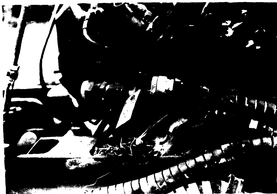
Figure 49. Tagged hydraulic fluid lines.
