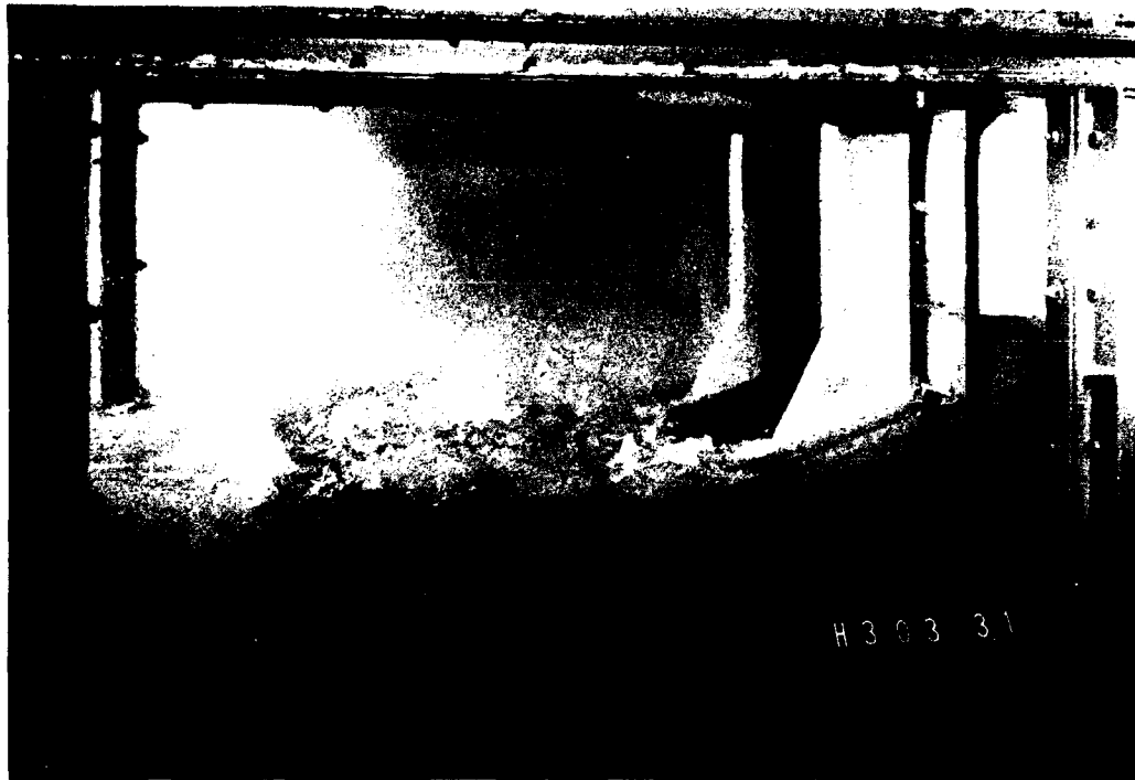
Photo 21. Hydraulic condition high bays = headwater el 30 ft, tailwater el 8 ft, gate opening 7.36 ft
