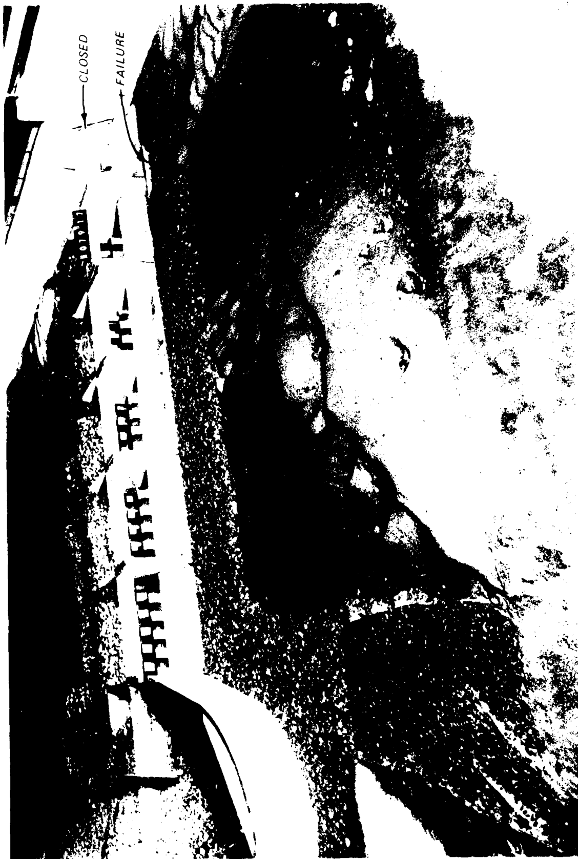
Photo 25. Areas of instability and scour potential, existing upstream riprap, five consecutive bays fully open, headwater el 68.0, tailwater el 56.0
