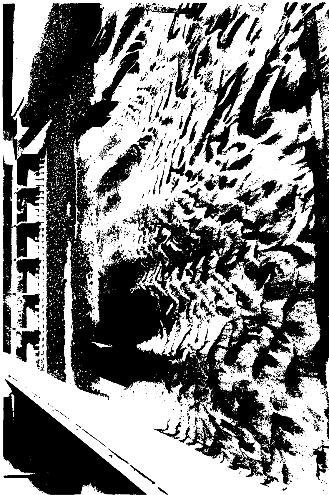
Photo 19. Areas of instability and scour potential, existing riprap, headwater el 62.0, tailwater el 52.0
