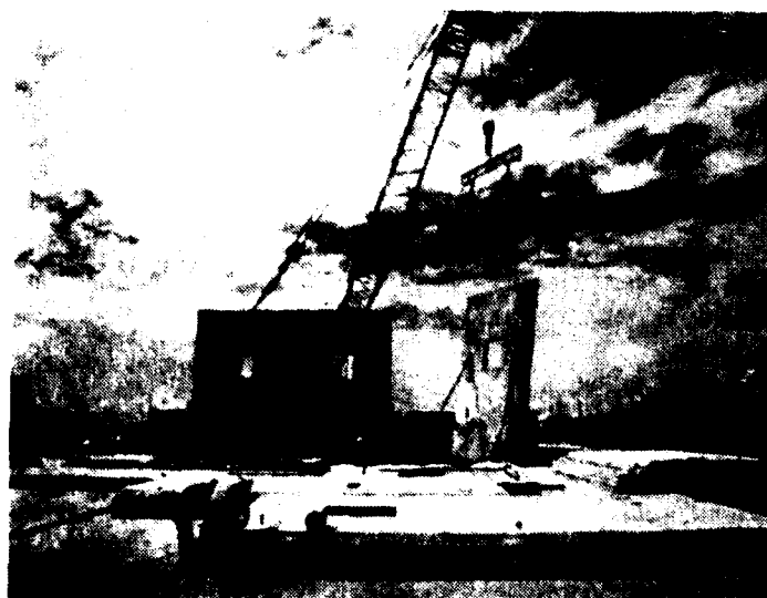
Figure 2. Precast concrete panel erection—Fort Bliss.
