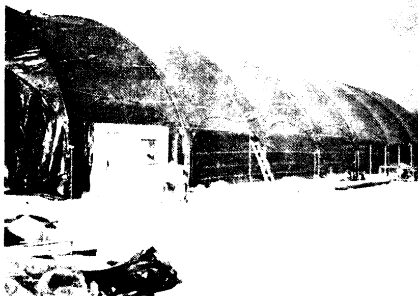
Figure 27. Installation of the fabric—Seoul.
