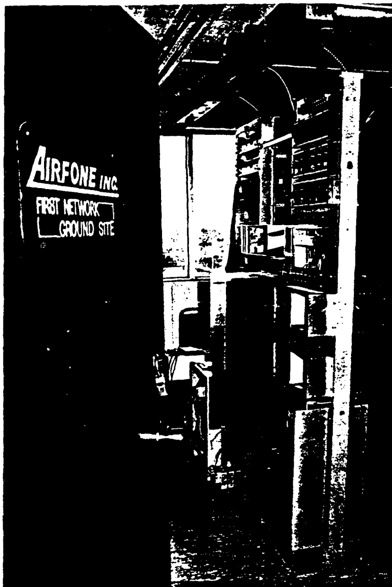
Figure 3-11 - Airfone Ground Station in Chicago 35
