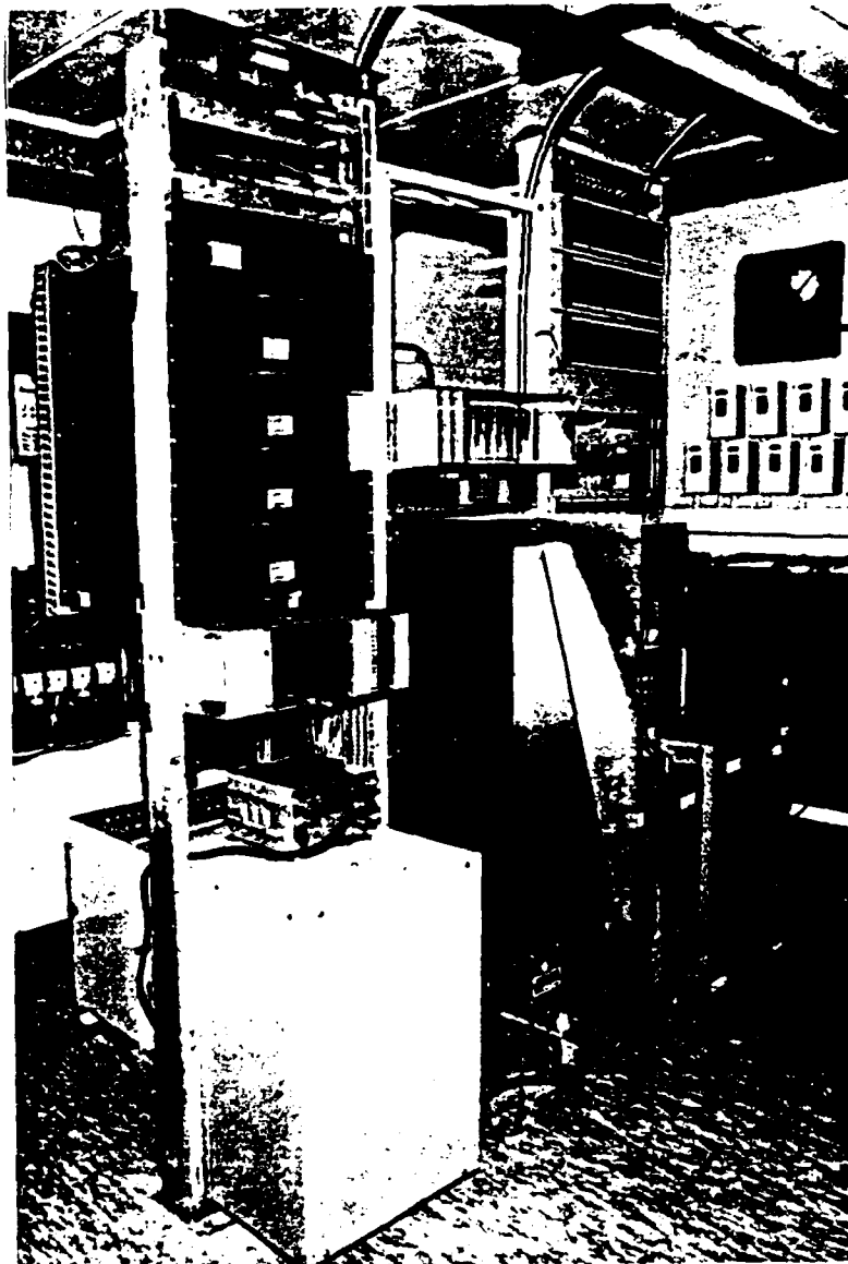
Figure 3-12 - Airfone Ground Station in Chicago 36
