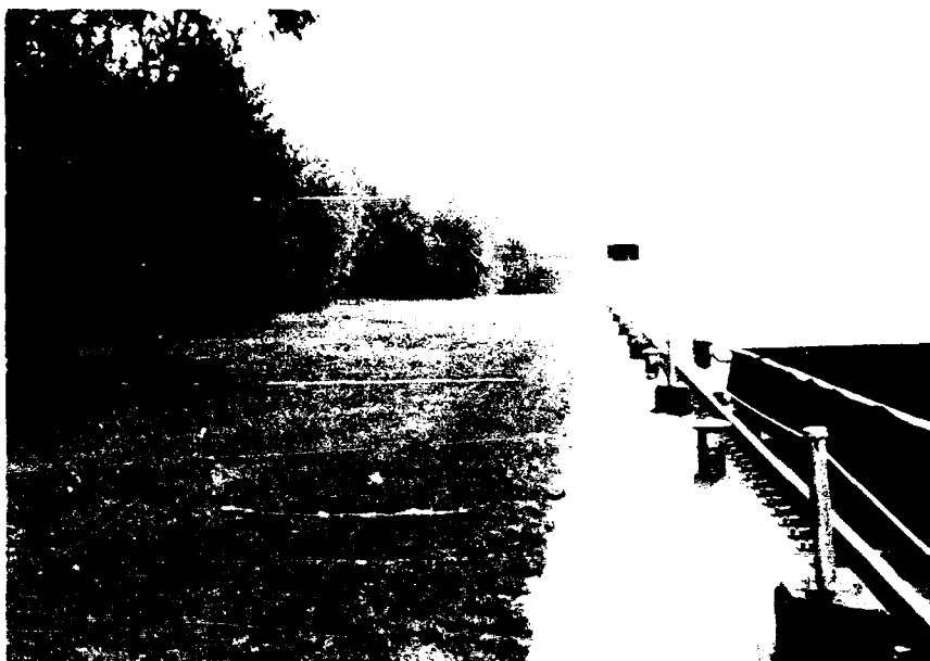
Figure 1. Grassed area behind upper guide wall
