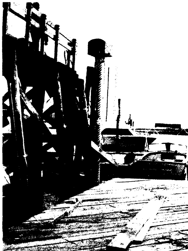
Figure 24. Installation of stilling well tidal elevation recorder at Town Dock
