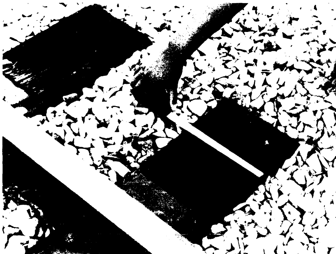
Figure 31. Measuring the top dimension of a tie.
