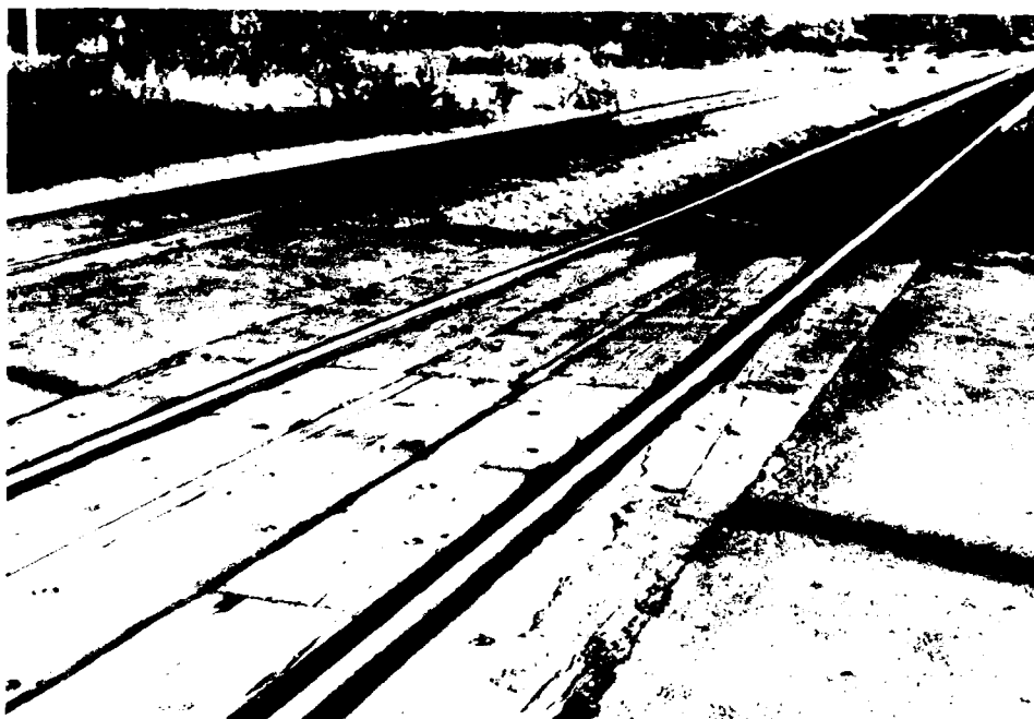
Figure 51. Timber road crossing.
