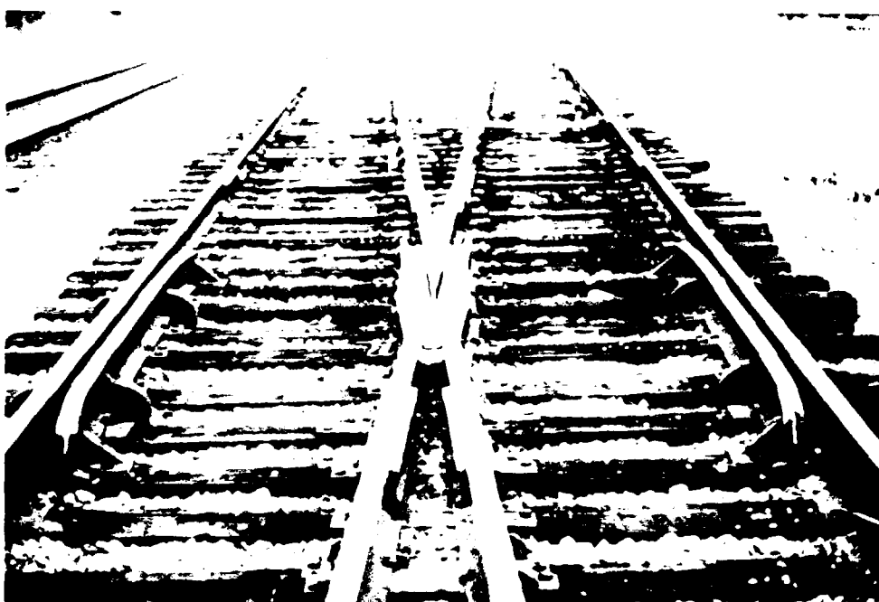
Figure 38. Rail-bound manganese (RBM) frog for turnout.
