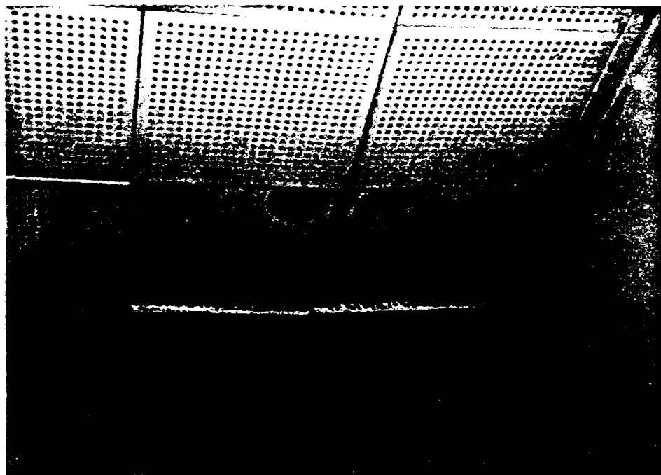
Figure 46. Ceiling crack in Room 104.
