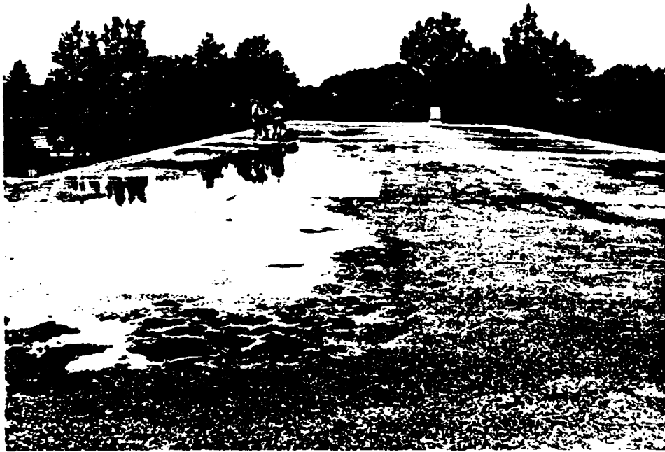
Figure 32. Poned water on south side of west wing.
