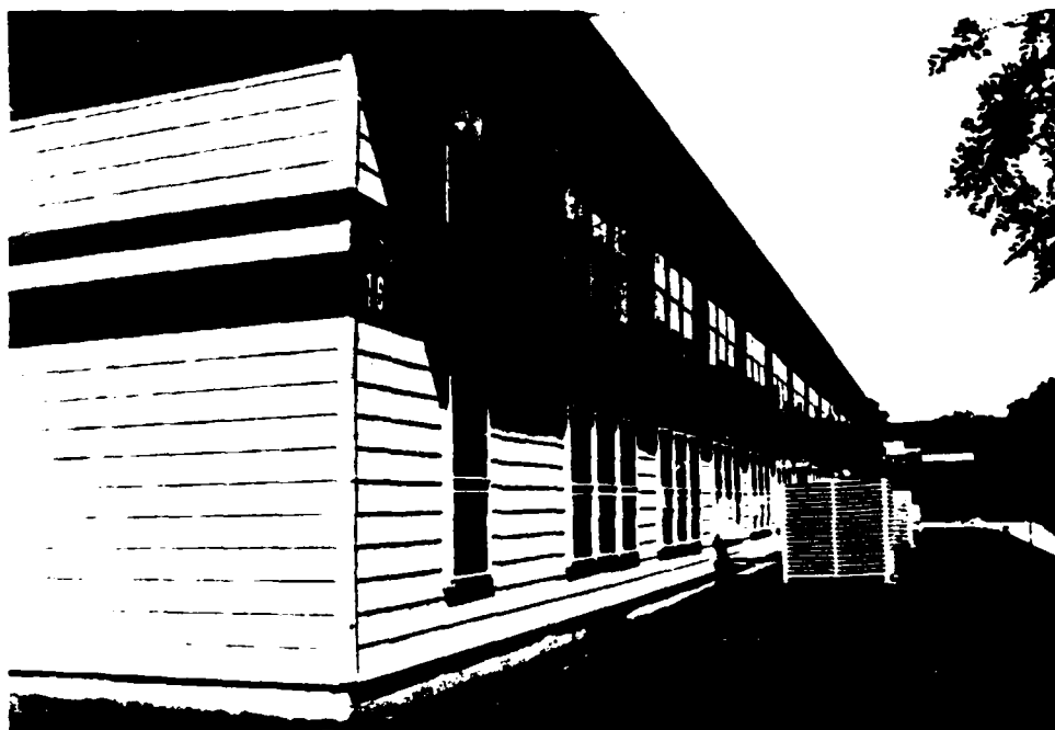
Figure 2. Building 16, west wing, south elevation.
