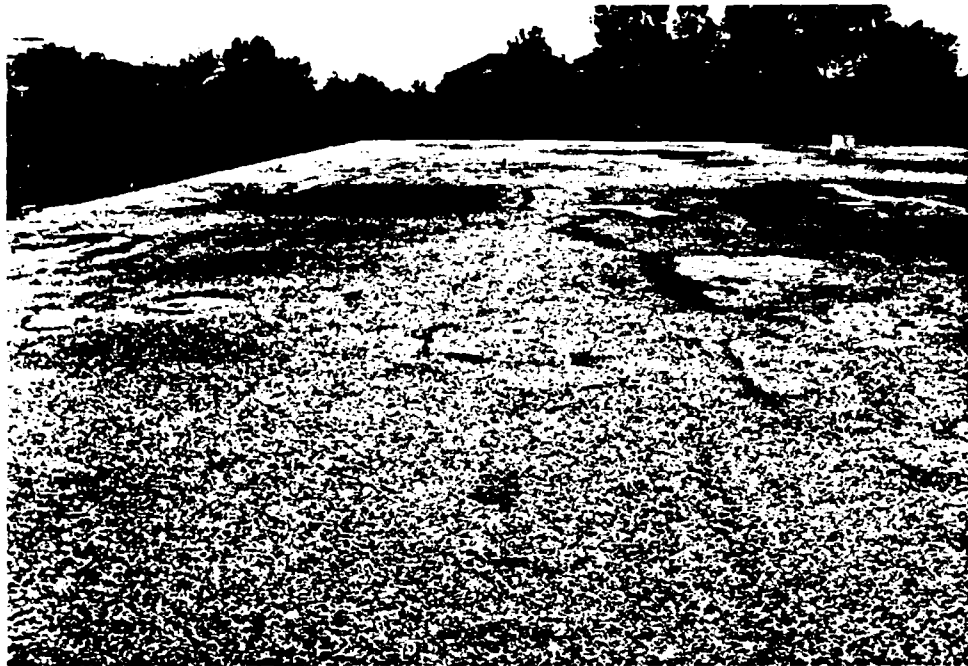
Figure 24. Several patches in roof surface.
