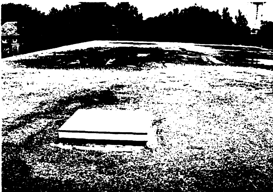
Figure 33. Poned water on west side of north wing.
