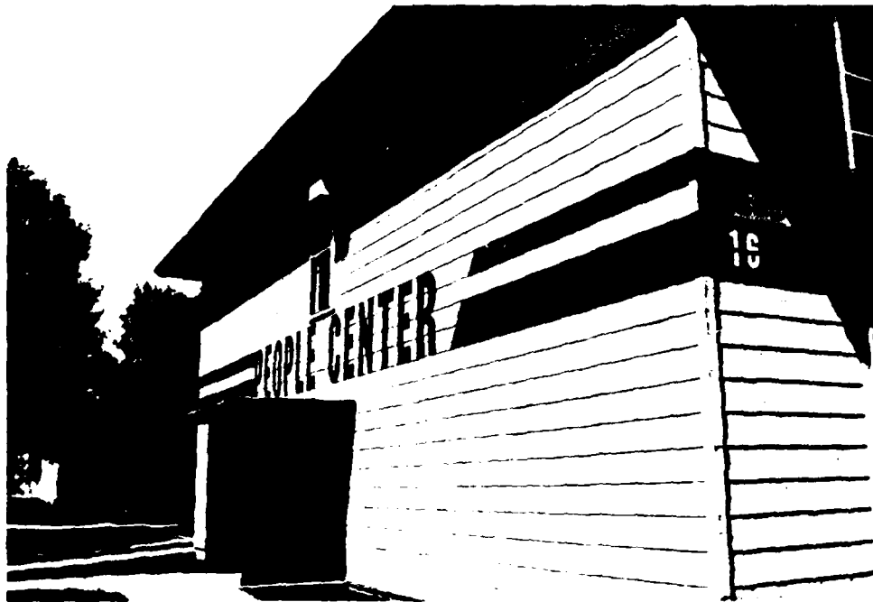
Figure 3. Building 16, west wing, west elevation.
