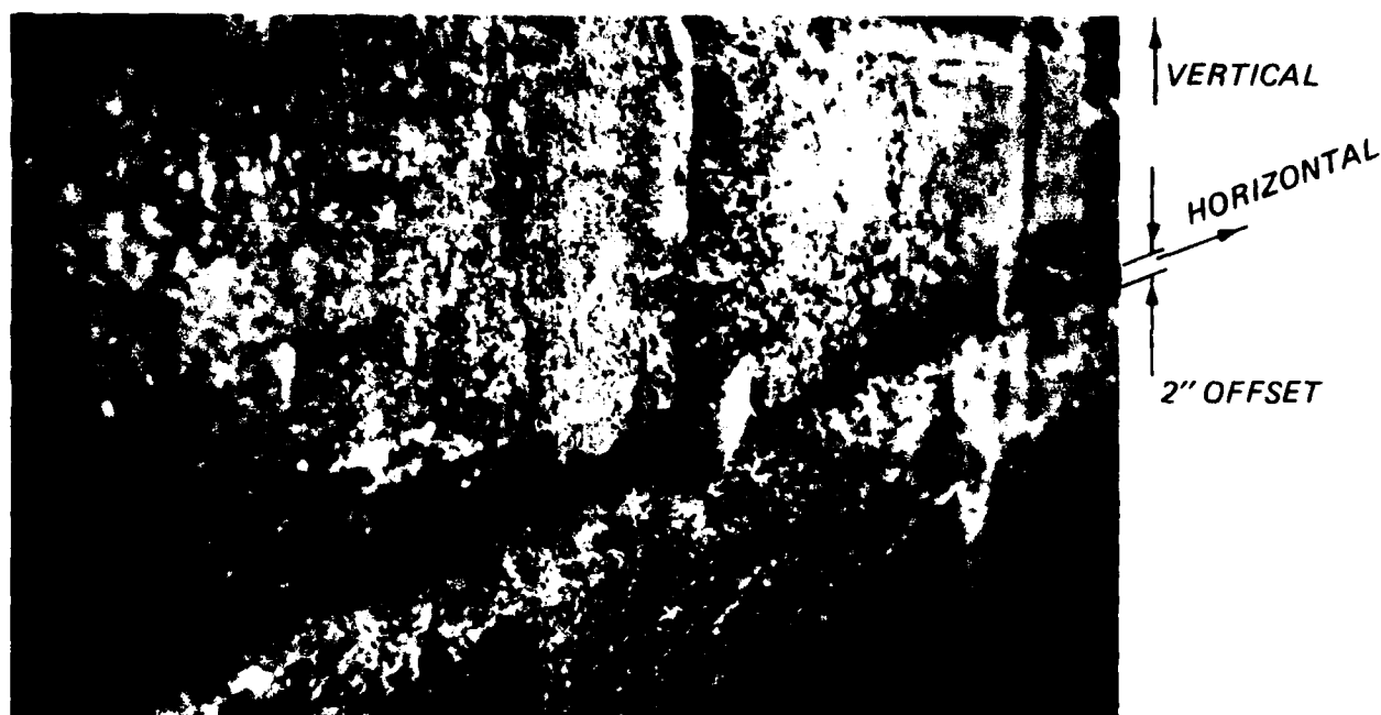
Figure 34. Photograph of offset (approx 2 in.) between concrete caissons in Quebec Harbor, Canada
