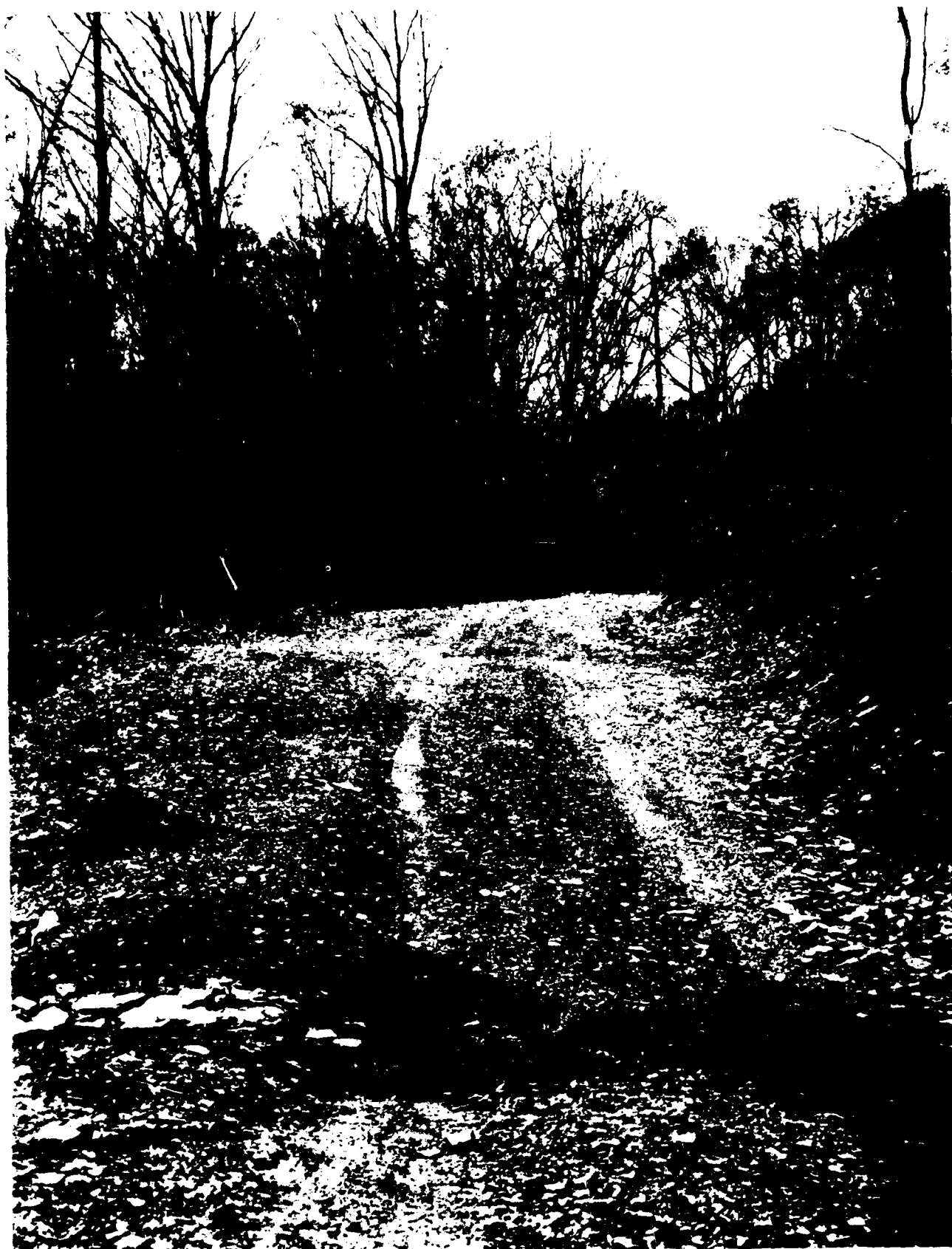
Figure 4.--The ungraveled section in Replication 3 showing the high coarse fragment content.
