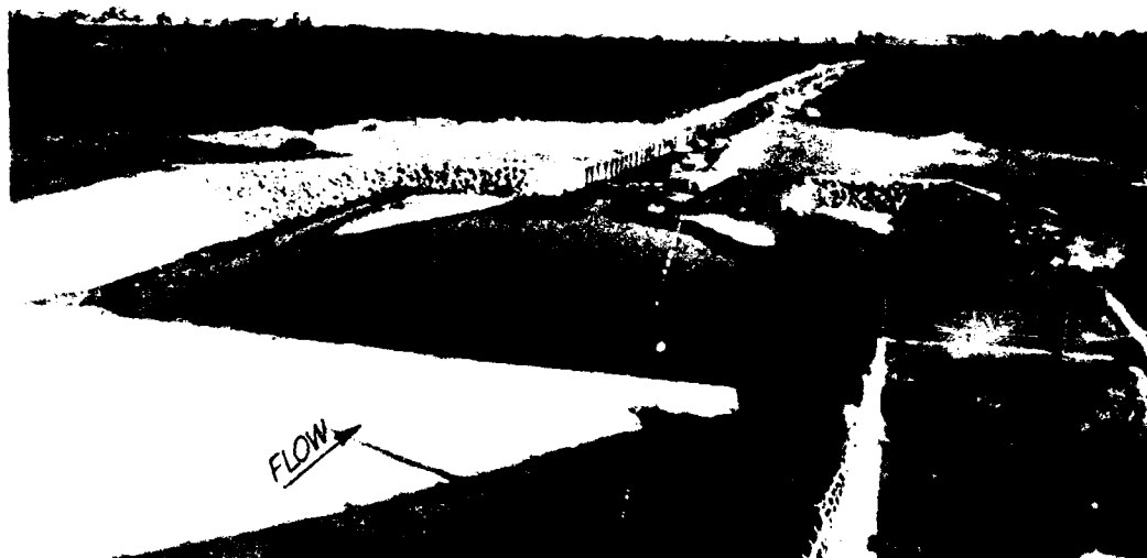
Figure 2. Stilling basin and Oak Street Drain downstream of the spillway.
