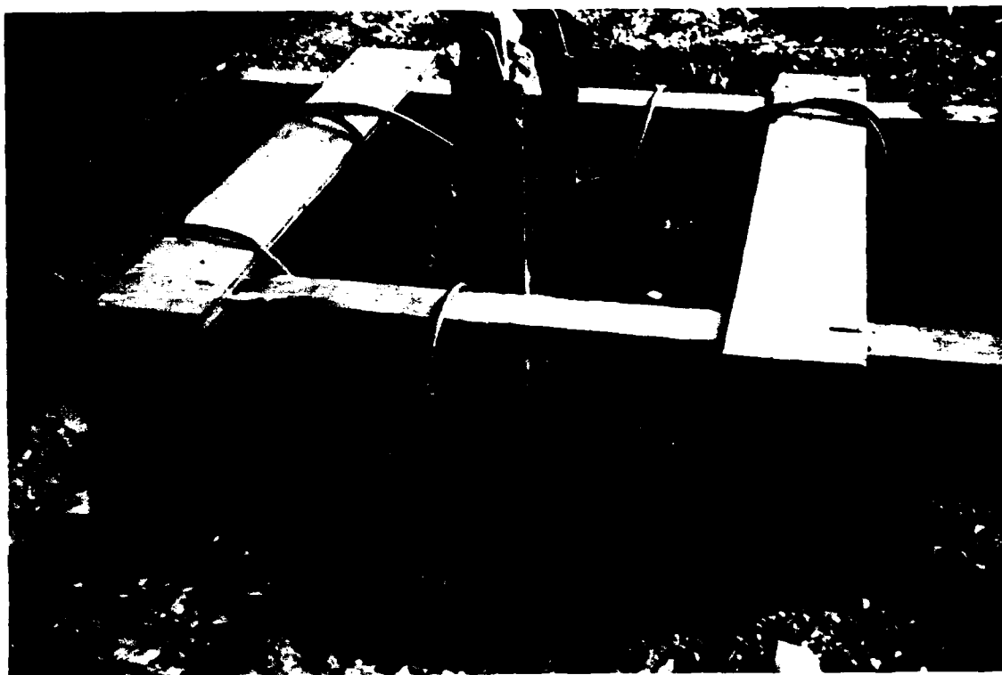
Figure B2. Thawing of frozen ground around the upper 3.7 m of the H-pile using steam thaw points prior to field calibration.
