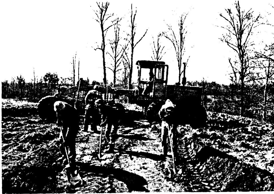
Figure 21. View of field crew cleaning motor grader transect, looking north.
