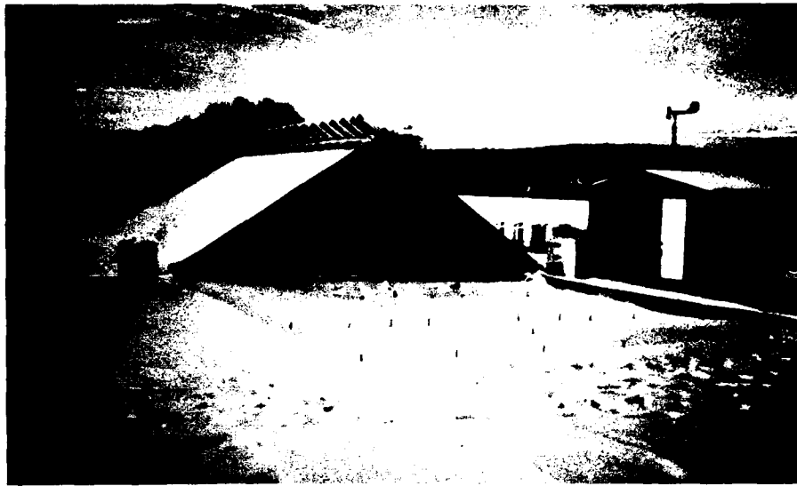
a. Snow-covered roof of bed with lattice work at gabled end.
